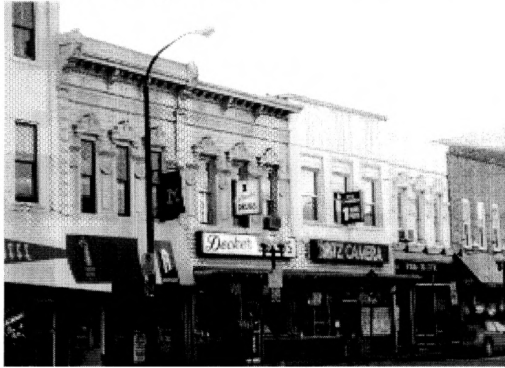
Fig. 6.12. Few varied but well kept storefronts on the West Facade. Source: Photograph by the Author.
