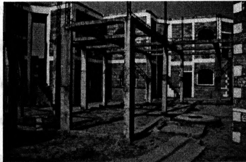
Figure 4.6 Close-up of the structural framework. (Note the use of slender prefabricated welded trussed girders as reinforcement-cheaper than conventional reinforcement).
