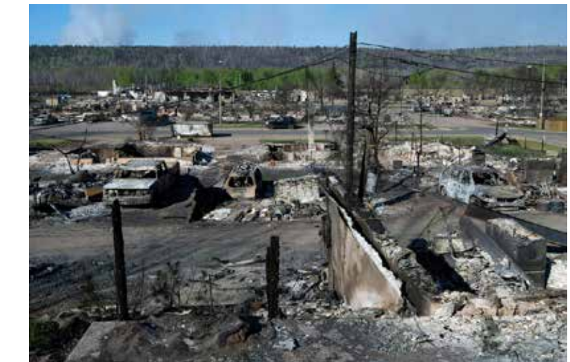
Figure 2.3. Fort McMurray neighborhood wildfire damage. [PremierofAlberta/Flickr. 2016. Used under Creative Commons.]
