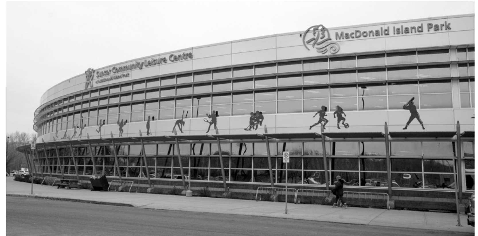
Figure 4.20. Multi-million dollar recreation facility for 50,000 people. [Author 2016]
