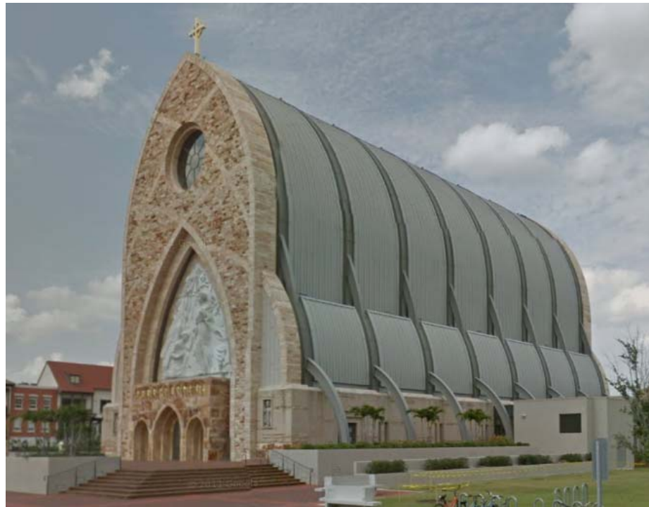
Figure 2-8. Southwest view of the Ave Maria University Oratory. Photo courtesy of (Google, 2017).
