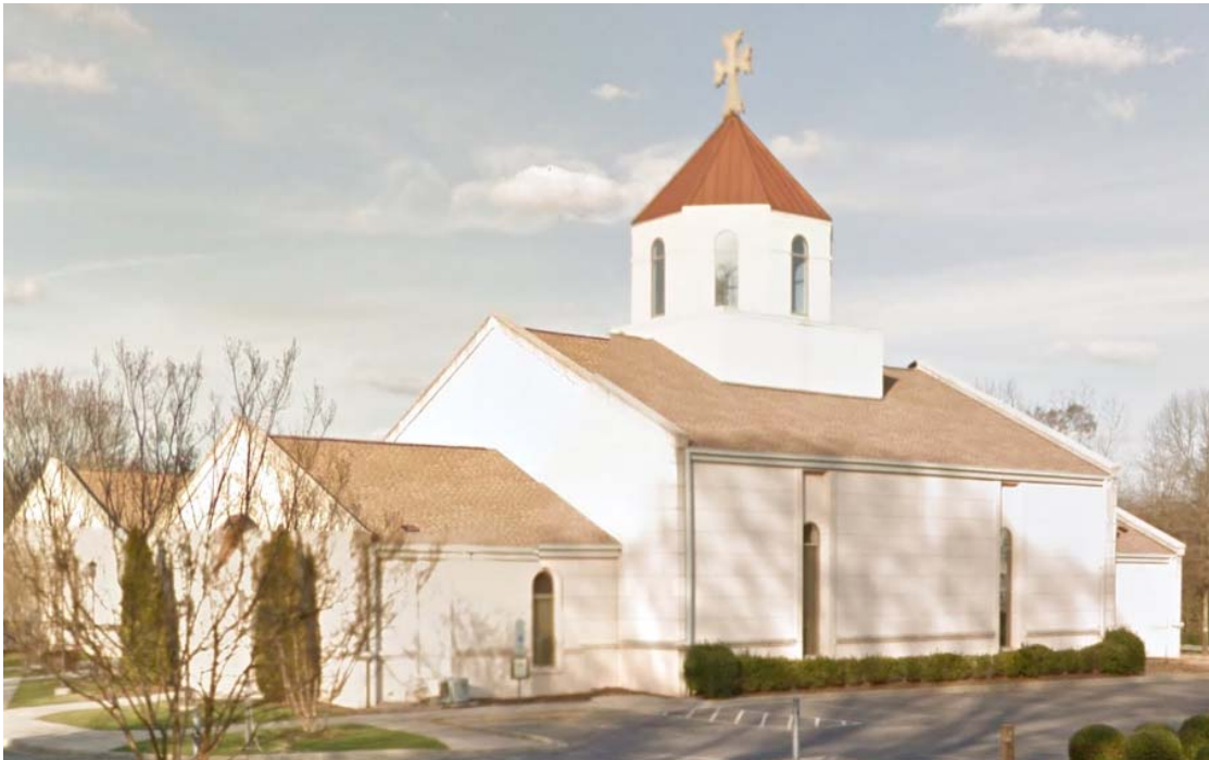
Figure 2-10. St. Sarkis Armenian Apostolic Church in Charlotte, North Carolina completed in 2005. Architecturally designed by SAA Architecture, LLC and constructed by Seretta Construction. Photo courtesy of (Google, 2017).
