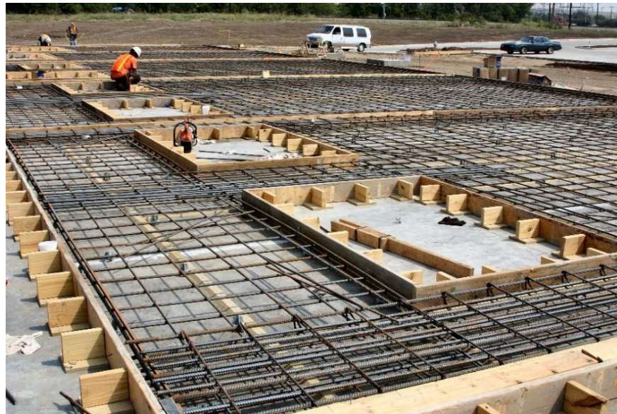
Figure 1-1. Formwork for casting the wall panel using dimension lumber. Photo courtesy of (constructionphotographs.com, 2012).
