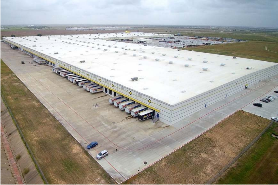
Figure 2-3. Southeast view of the Room To Go Distribution/Showroom in Brookshire, Texas. Photo courtesy of (Bob Moore Construction, 2014).
