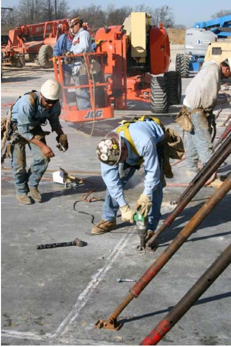
Figure 1-4. Braces screwed onto the slab. Photo courtesy of (constructionphotographs.com, 2012).
