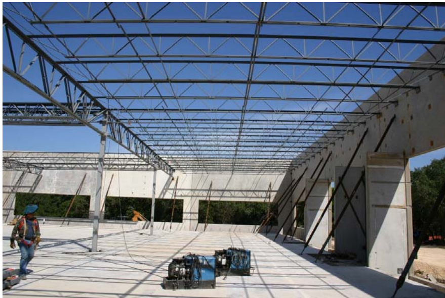
Figure 1-3. Roof framing installed after wall panels are in place. Photo courtesy of (constructionphotographs.com, 2012).
