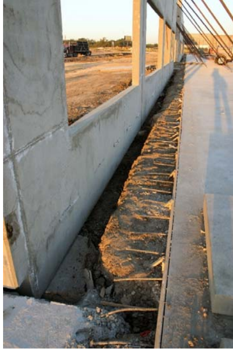
Figure 1-2. Tilt-up wall panels positioned on footing pads. Photo courtesy of (constructionphotographs.com, 2012).
