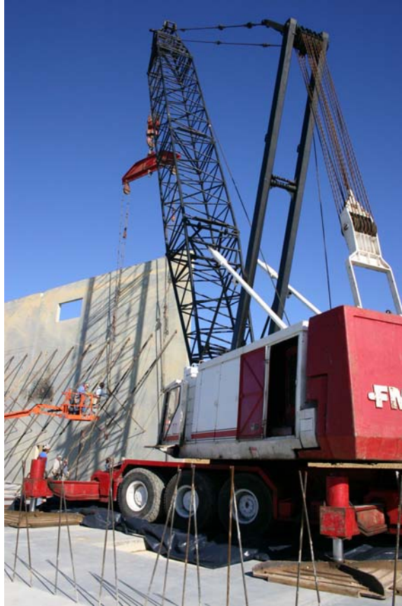
Figure 4-1. Truck crane with outriggers on the slab. Photo courtesy of (constructionphotographs.com, 2012).
