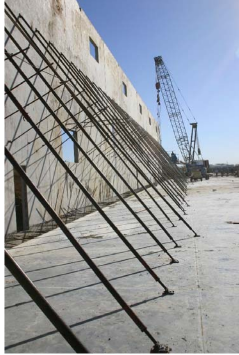
Figure 1-5. Tilt-up wall panel bracing. Photo courtesy of (constructionphotographs.com, 2012).
