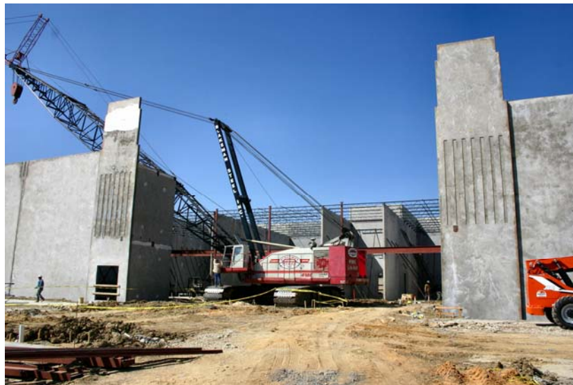
Figure 4-2. Crawler crane off the slab. Photo courtesy of (constructionphotographs.com, 2012).
