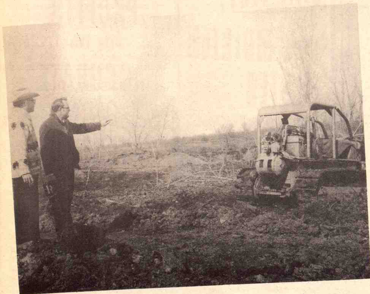
START OF LEVELING Dr. Robert Hyde, Extension range and pasture specialist from KSU, and Bill Cox, Crawford county Extension agricultural agent, watch as bulldozer levels strip mined land.
