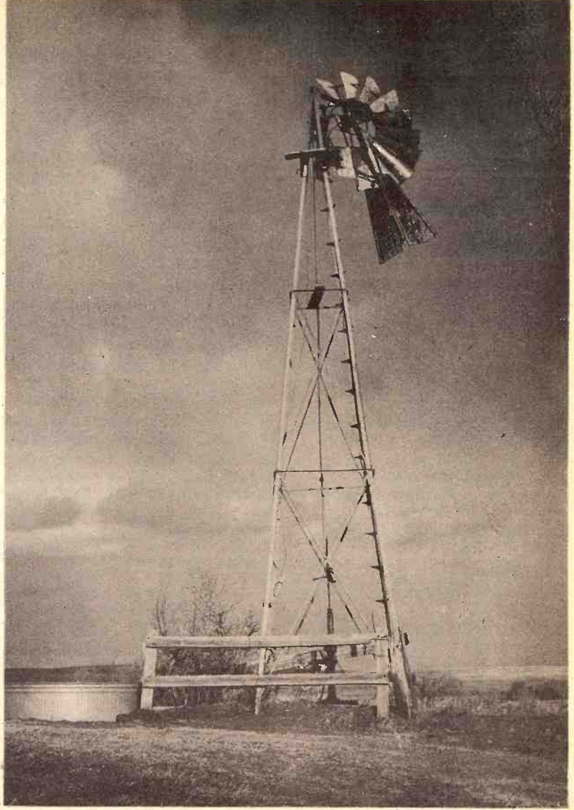
SYMBOL OF WIND DAMAGE Symbolic of recent storm damage to ranchers and farmers in the Grass & Grain area is this broken windmill near Tescott.
