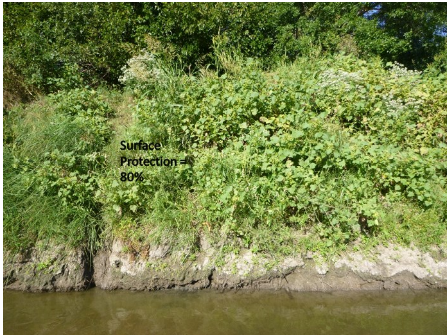
Figure 2.10 Surface Protection Example – Lower Little Arkansas River Study Bank #2
