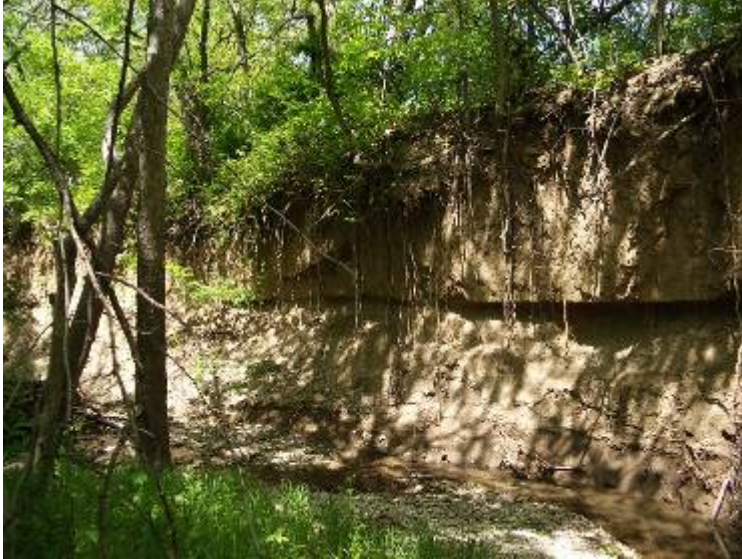
Figure 5 - Severly entrenched section of Little Kitten Creek. [Source: authors personal collection]
