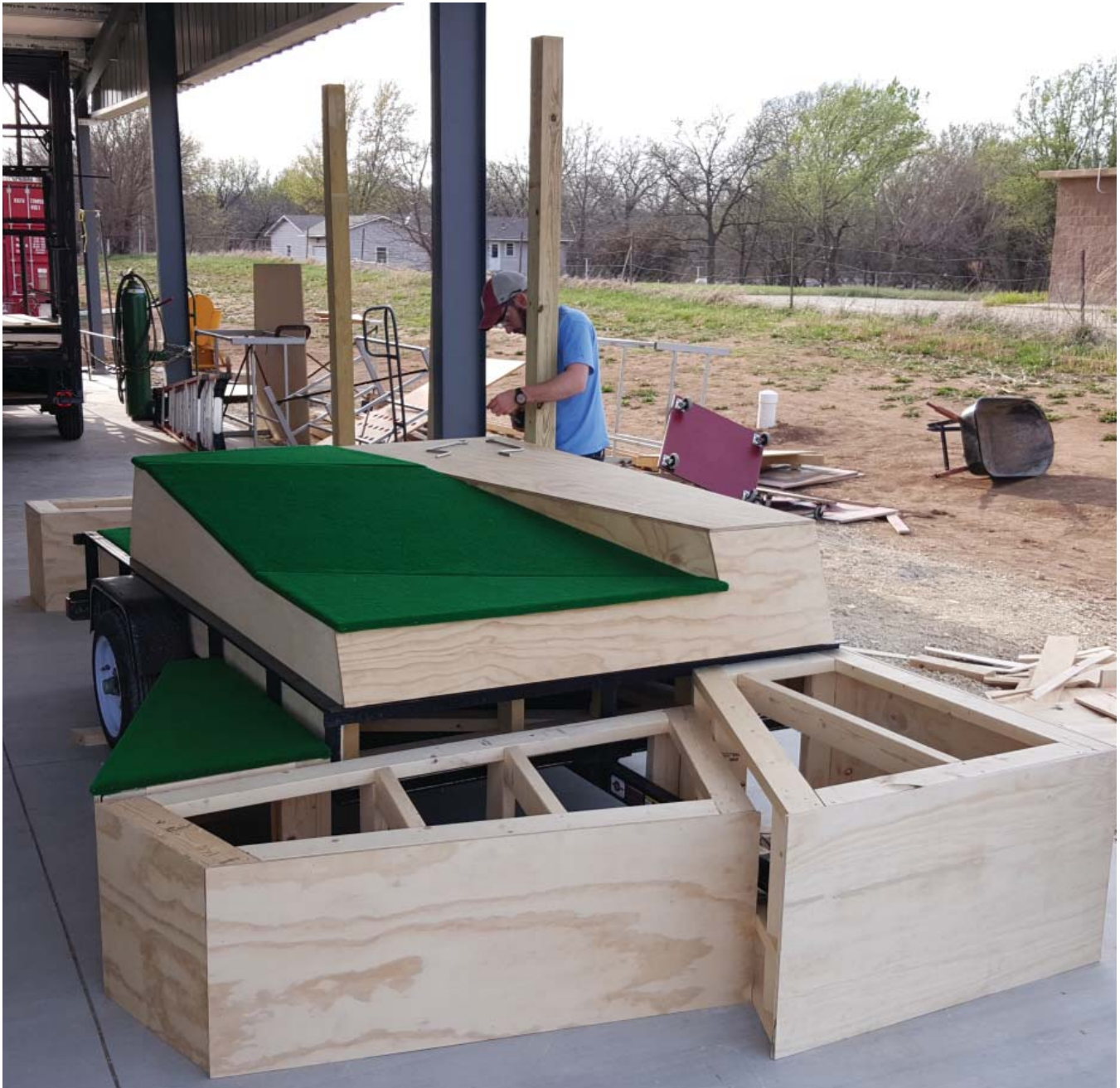
Figure 5.46: Constructing Portable Landscape Prototype (Borwege 2016)
