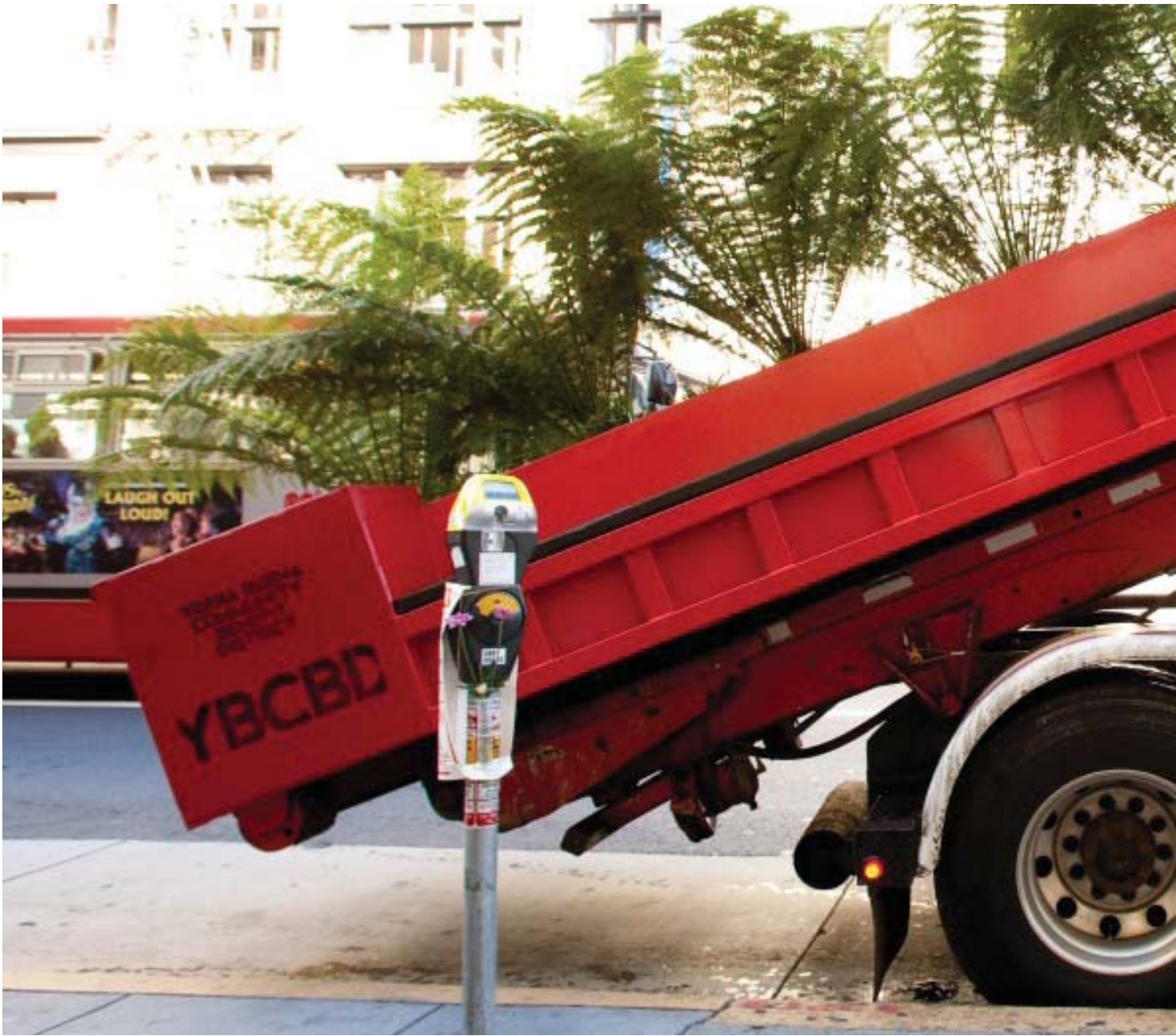
Image 4.10: Transporting and Installing Parkmobile (CMG Landscape Architecture 2011)
