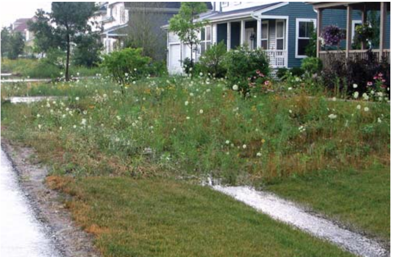
Figure 3.18 Prairie Crossing-Bioswale. By AES
