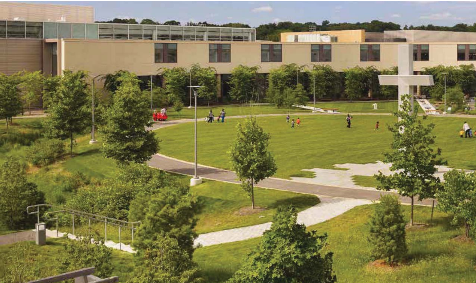
Figure 3.20 The Ray and Joan Kroc Corps Community Center-Aerial View. By AA
