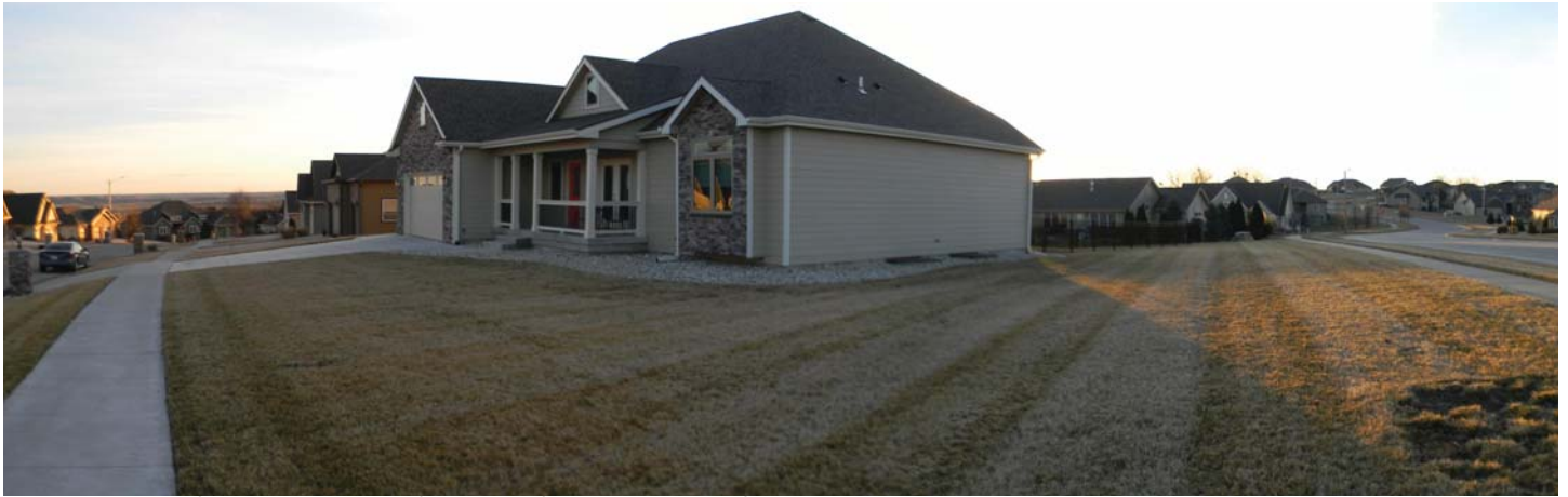
Figure 5.10 East Park Grove Drive Frontyard Facing Southwest-View A. By Author
