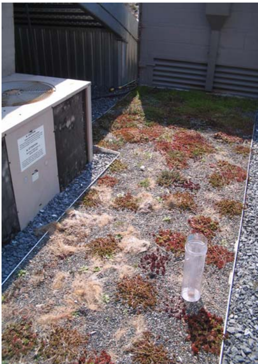
Figure 2.25 North Terrace with Stormwater Gauge.
