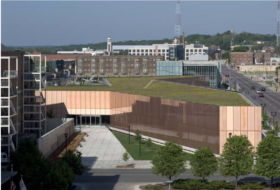
Figure 2.35 Completed Green Roof and Library (Kain, 2007).
