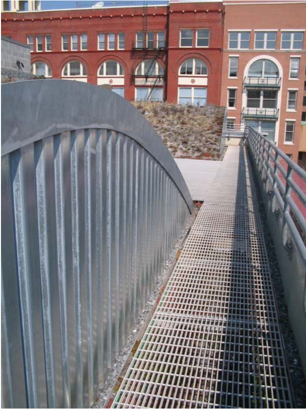
Figure 2.22 Steel Railing and Side of South Wave.
