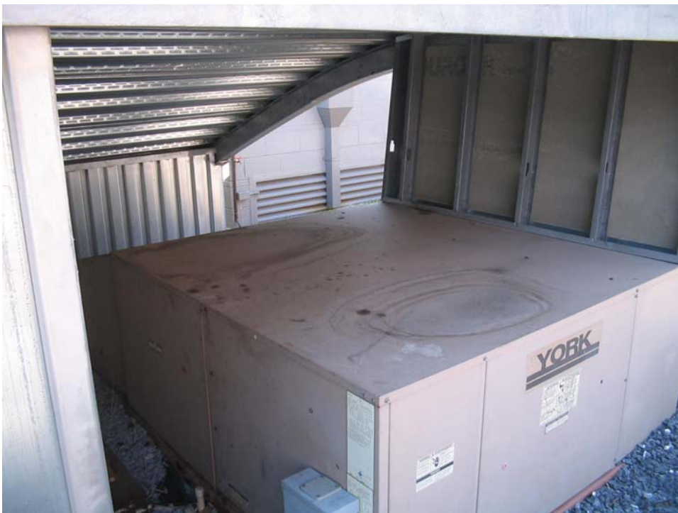
Figure 2.27 HVAC Under North Wave.
