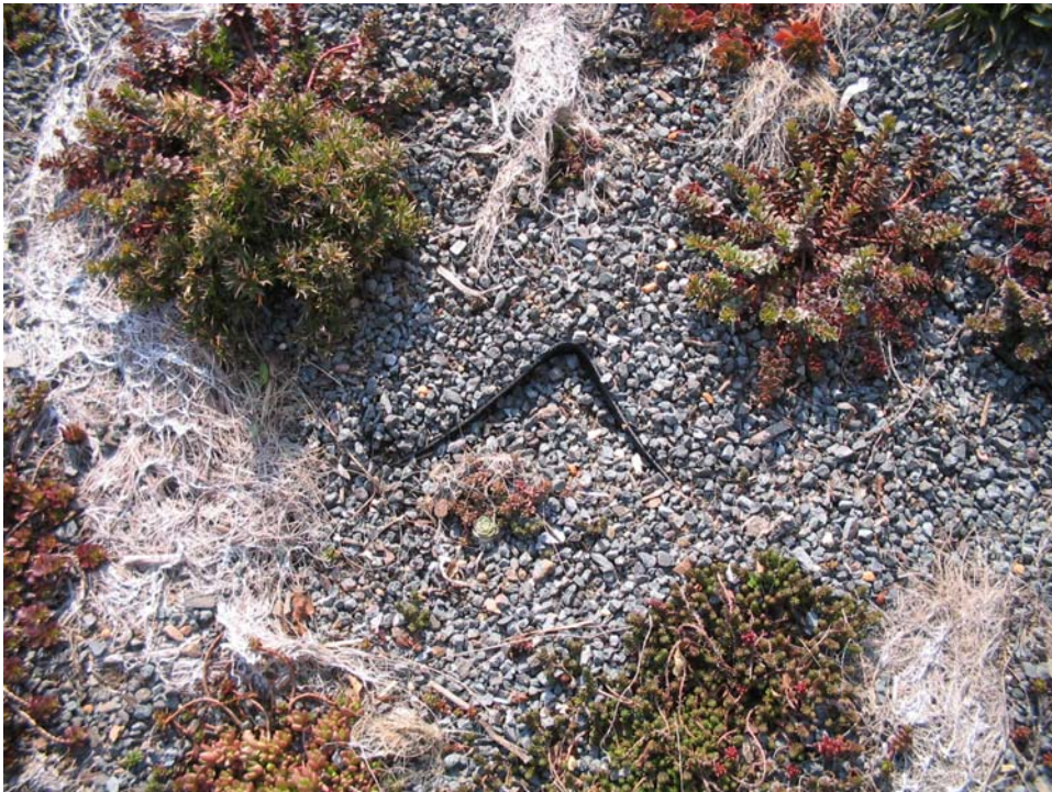
Figure 2.31 Exposed Vinyl Soil Stabilization System.
