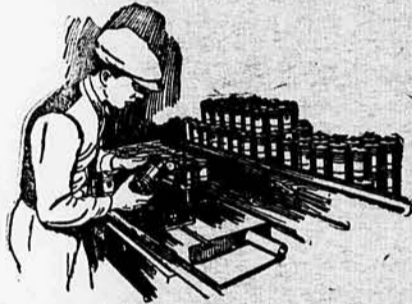
Inspecting a finished piston with dial-faced gauge that measures to the thousandth part of an inch.
