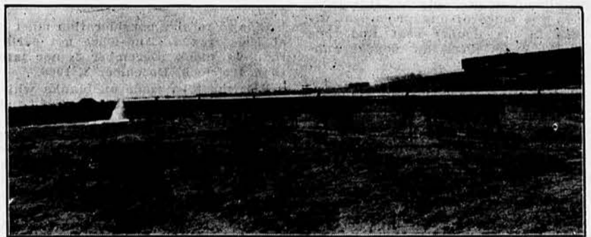
Line of pipe conveying the beet "pomace" from the Garden City Beet-Sugar factory to the large earthen "silo." Sugar-beet pomace in foreground.
