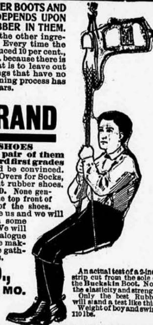
An actual test of a 2-inch strip cut from the sole of the Buckskin Boot. Note the elasticity and strength. Only the best Rubber will stand a test like this. Weight of boy and swing 110 lbs.
