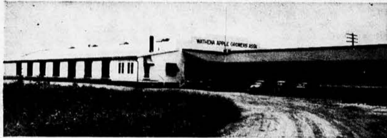
STORAGE: Here is packing shed and cold-storage plant owned by the Wathena Apple Growers Association, at Wathena. Combined capacity will take care of 40,000 bushels.
