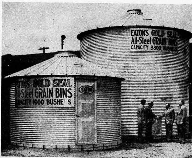
The Eaton Metal Products Co., Omaha, announces several improvements in their all-steel galvanized grain bin models, which run from 1,000- to 3,000-bushel sizes. Improvements include a one-piece pressed door for greater strength; a redesigned door frame to make the door watertight; a new one-piece ventilator top, and improved fabricating methods that provide tighter joints between side sheets.
