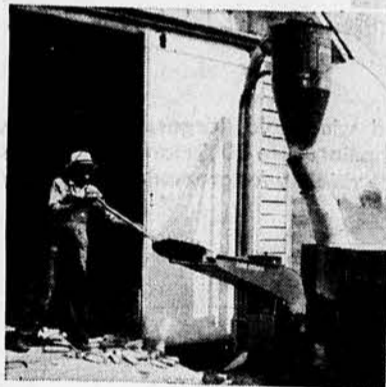
At Right: The John Deere No. 114-A Roughage Mill. The big-capacity traveling feed table is governor-controlled for smooth, even feeding.
