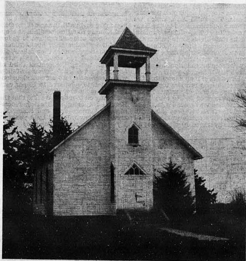
Front view of the Palestine Methodist church, Sumner county, Kansas. Built in 1914 and being moved this spring to Belle Plaine. The Palestine congregation and church building are being incorporated into the Belle Plaine church. (Photo by Harold Shankland, Kansas State College Extension Service, Manhattan.)
