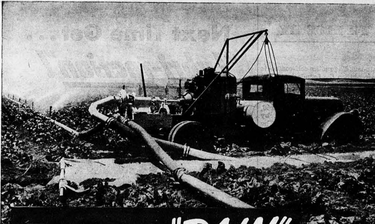
This portable overhead irrigation system, powered by a 3-cylinder GM Diesel engine, puts down one inch of water per hour over an area 1700 feet long by 120 feet wide.
