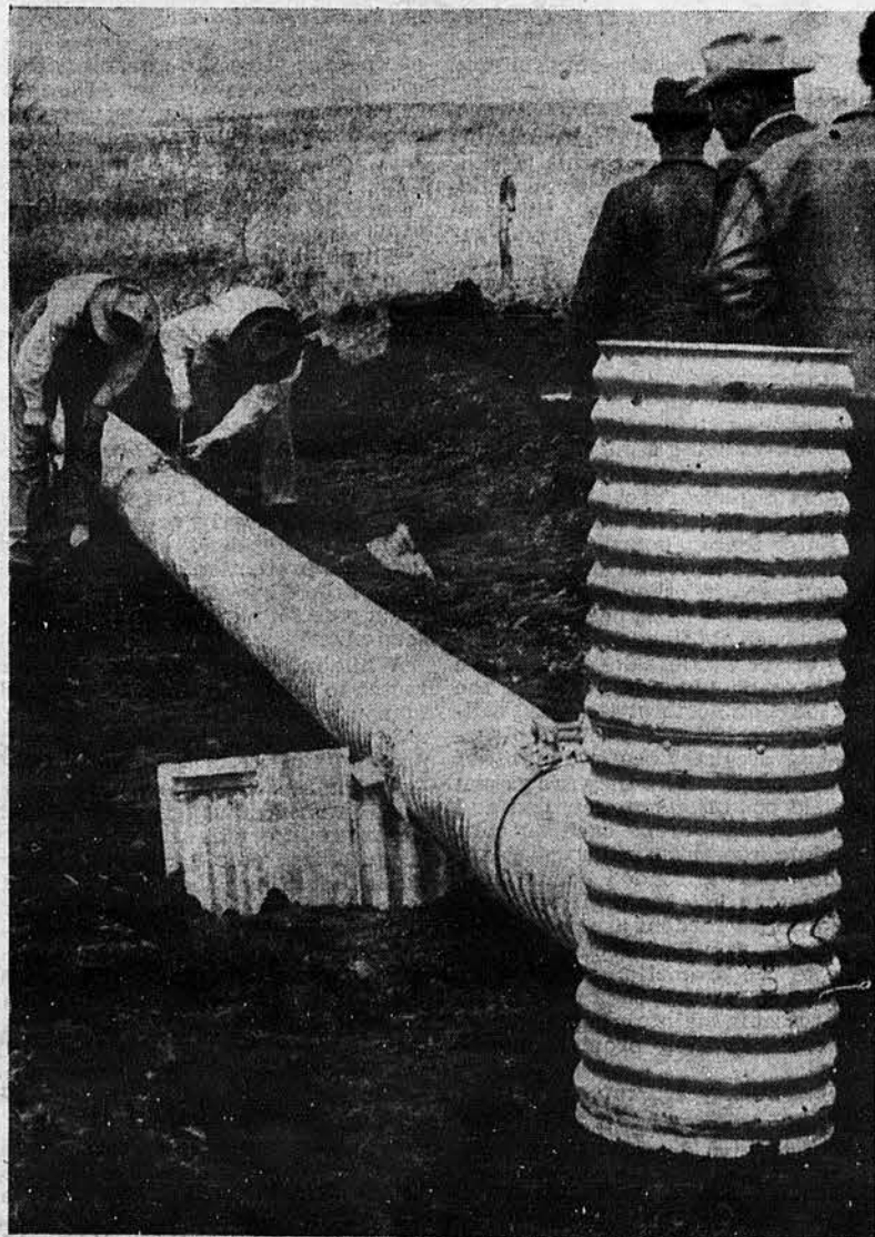
In a Shawnee county soil-conservation field day, April 19, farmers watched experts demonstrate how to install a tube and riser for a soil-saving dam. They also saw terrace building, waterway preparation, ditch filling, liming and fertilizing, seedbed preparation and actual seeding of legumes and grasses—all in one day on 3 farms.
