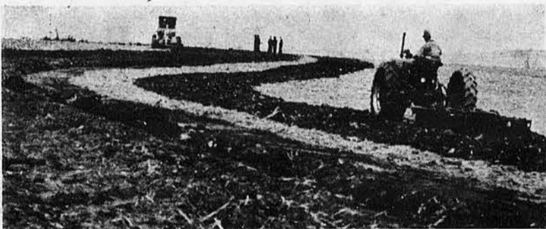
Almost every type of terracing equipment was used April 19, in Shawnee county, to completely terrace 3 farms in one day. The terraces shown here were built with a township road maintainer, left rear, while a tractor and disc worked the area between terraces.
