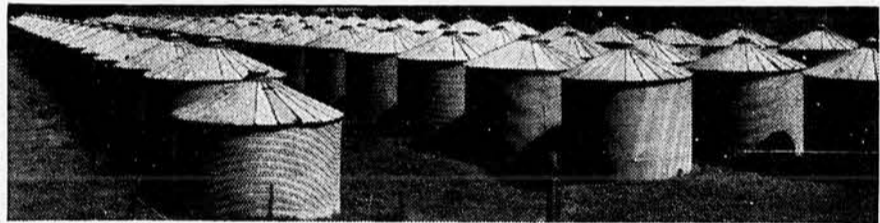
Pictured above is the U. S. Department of Agriculture installation of Eaton All Steel Grain Bins at Tekamah, Nebraska.
