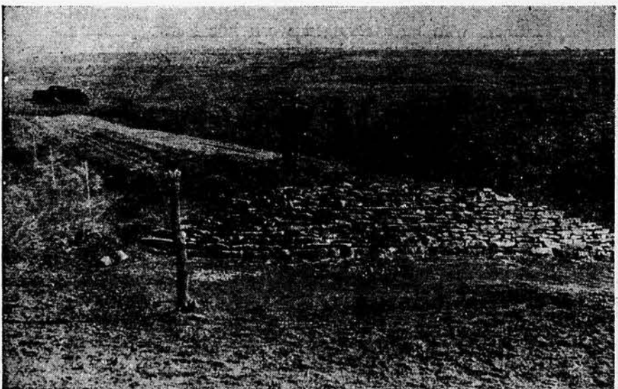
Proper riprapping of the spillway end of the dam, like this one on the Fred Krug farm, in Osborne county, will help insure your investment in a good dam. Note the fencing.
