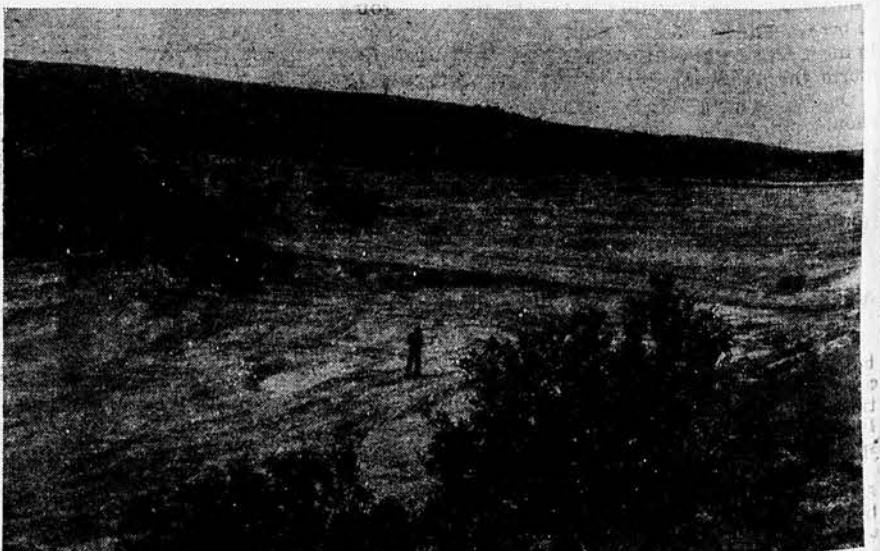
This dam, in Rooks county, contains 6,000 yards of dirt and will impound about 25 acre-feet of water. It is one of 2 such dams recently constructed by Leo Dreiling.
