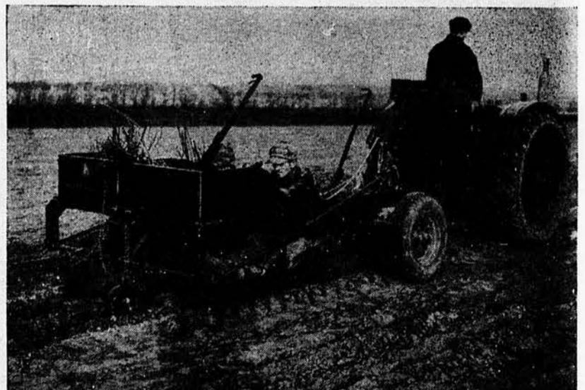
Tree-planting machine developed by the Forest Service of the U. S. Department of Agriculture. One machine will plant from 800 to 1,000 trees an hour.
