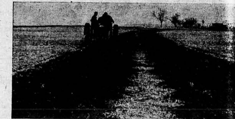
A scene on the Hampton Shirer farm, Geary county, showing a plowed terrace under construction. Note unplowed ridge in the middle, which will be built up by deep plowing loose and unplowed soil toward center-line stakes.
