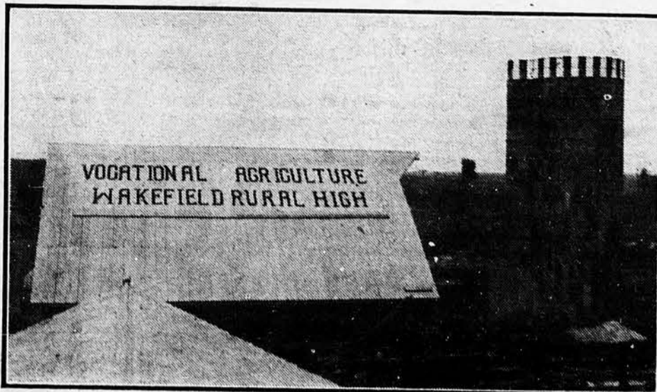
If one of the hens should perch on top of the laying house, this is the view she would get of the rest of the lay-out. The new silo is all complete except a cover over the ante-room in front.
