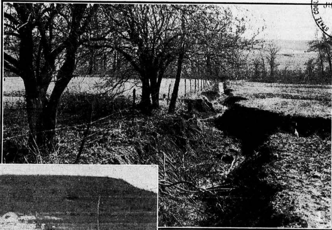
Above: A badly gullied outlet channel on a Montgomery county farm. Terraces emptying down this fence line from each side caused the ditch. The men are standing back from the outlet channel, where water has cut out the base of terrace channels.
