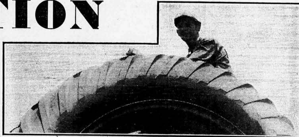
Above, rolling along on air and water. H. F. Roepke, Pottawatomie county, has each of the big tires filled two-thirds full of water. This extra weight increases the ground traction and results in more power.
