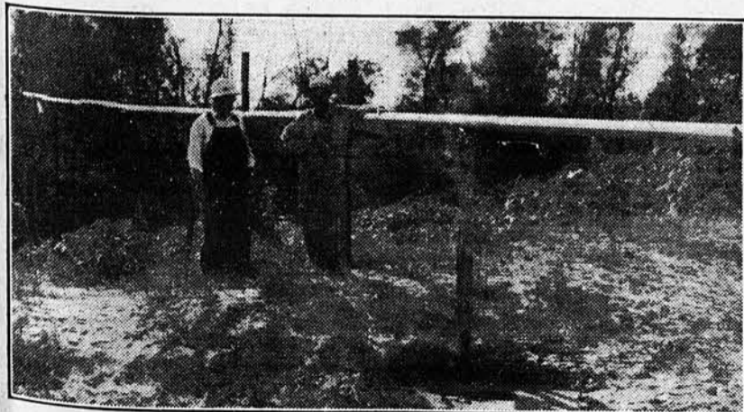
A. S. Parr and Howard Stiles, Rossville, at Mr. Stiles' irrigation plant south of town. This shows how water can be carried back to the farming land cheaply by means of lightweight pipe. Mr. Stiles irrigates melons, tomatoes and many vegetables.
