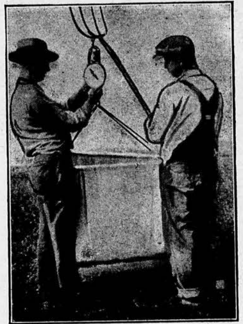
Alfalfa Yield Being Determined by County Agent M. C. Axelton, Yates Center, in Variety Test on the J. S. Marks Farm. A Canvass Sling, Suspended on a Pitchfork, Holds the Hay. A Spring Scale Is Used
