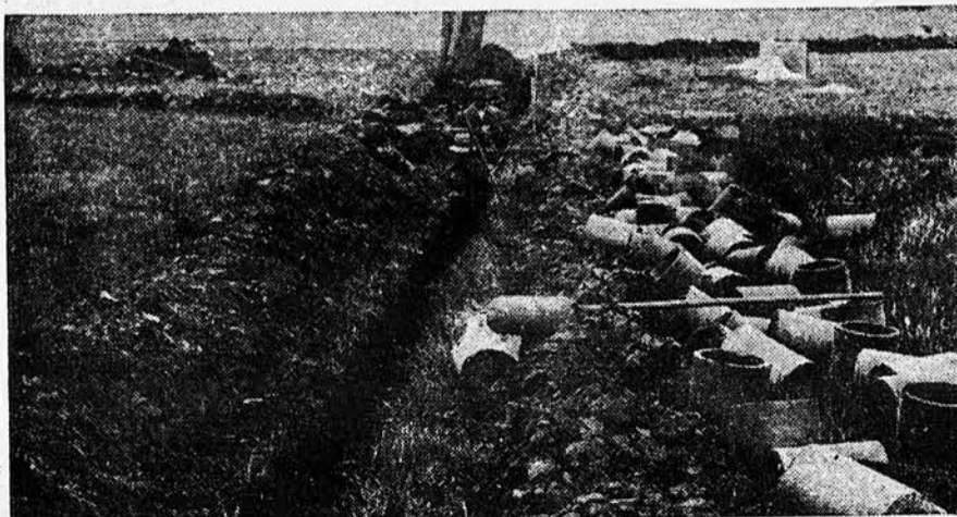
More Tile Drainage is Required in Kansas, as the Big Damage from the Excessive Moisture in 1915 Quite Well Demonstrated.
