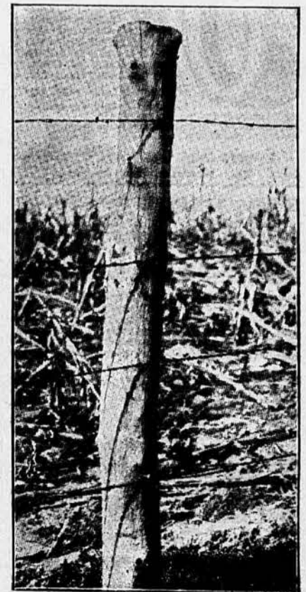
This is a Treated Ash Post Set 10 Years Ago.
