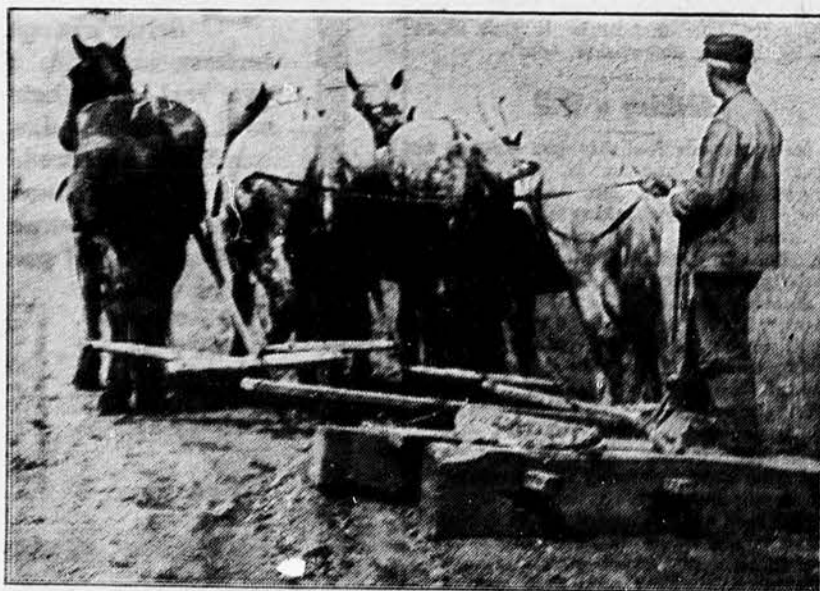
The Drag Should be Used as Soon as Possible After Rains as the Soil is in the Best Condition at This Time.
