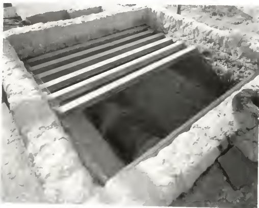
Figure 6B. Oil-Drum Flue in Trench Beneath Drying Floor Logs.
