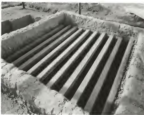
Figure 5B. Log Supports for Drying Floor
