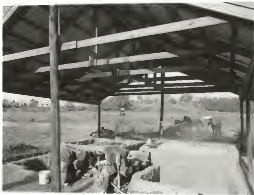
Figure 5A. Protective Shelter over Dryers
