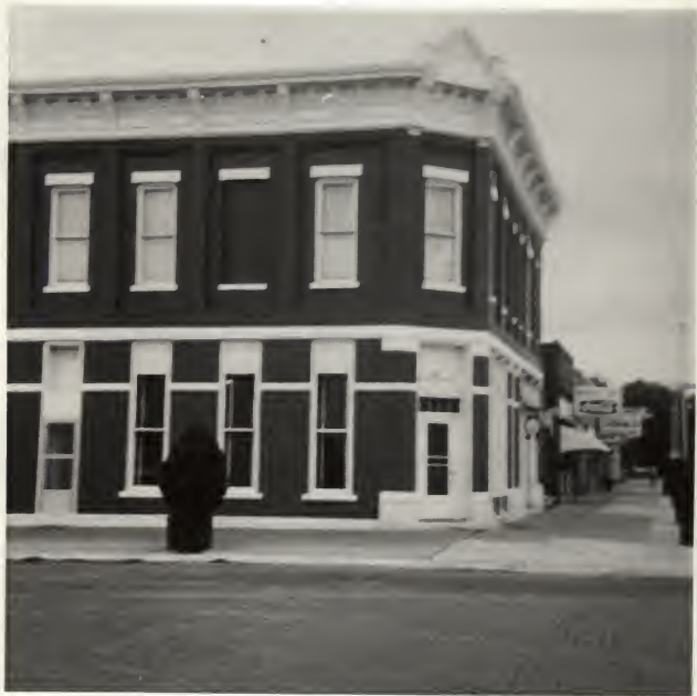
PLATE VII: A LINTSBORG STORE RENOVATION
