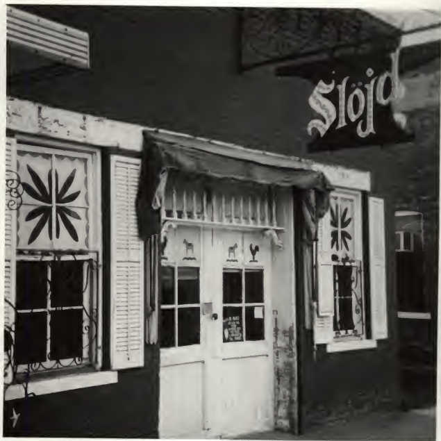
PLATE VI: A LINDSBORG STORE RENOVATION
