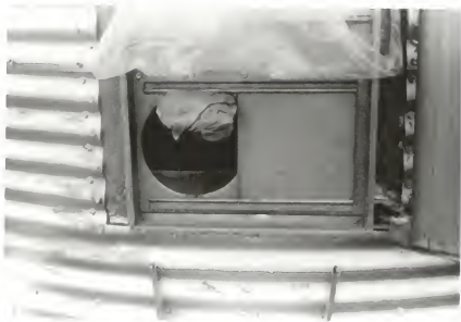
Figure 3.-Top - Drainage pipe attached to bin floor. Bottom - Drainage pipe coming out of the unload opening in the side door.
