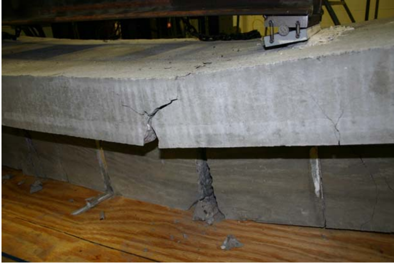
Figure 6.35 Failure for TB specimen
