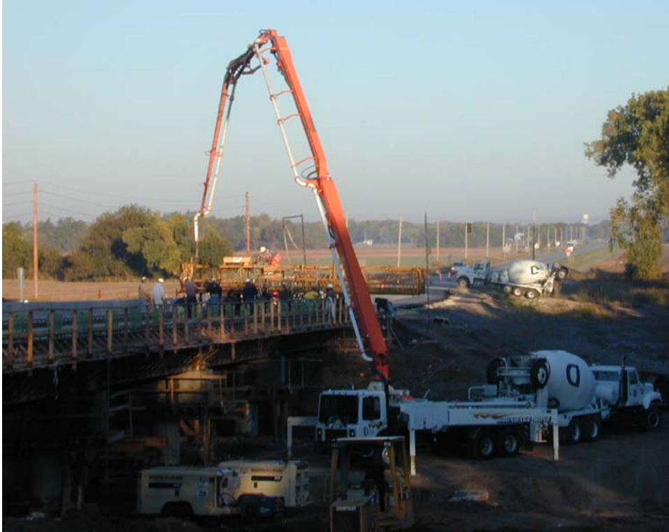
Figure 12.35 Pump truck for pumping concrete to bridge deck
