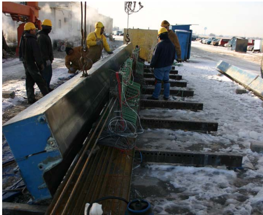
Figure 8.7 Side-form placement for IT600
