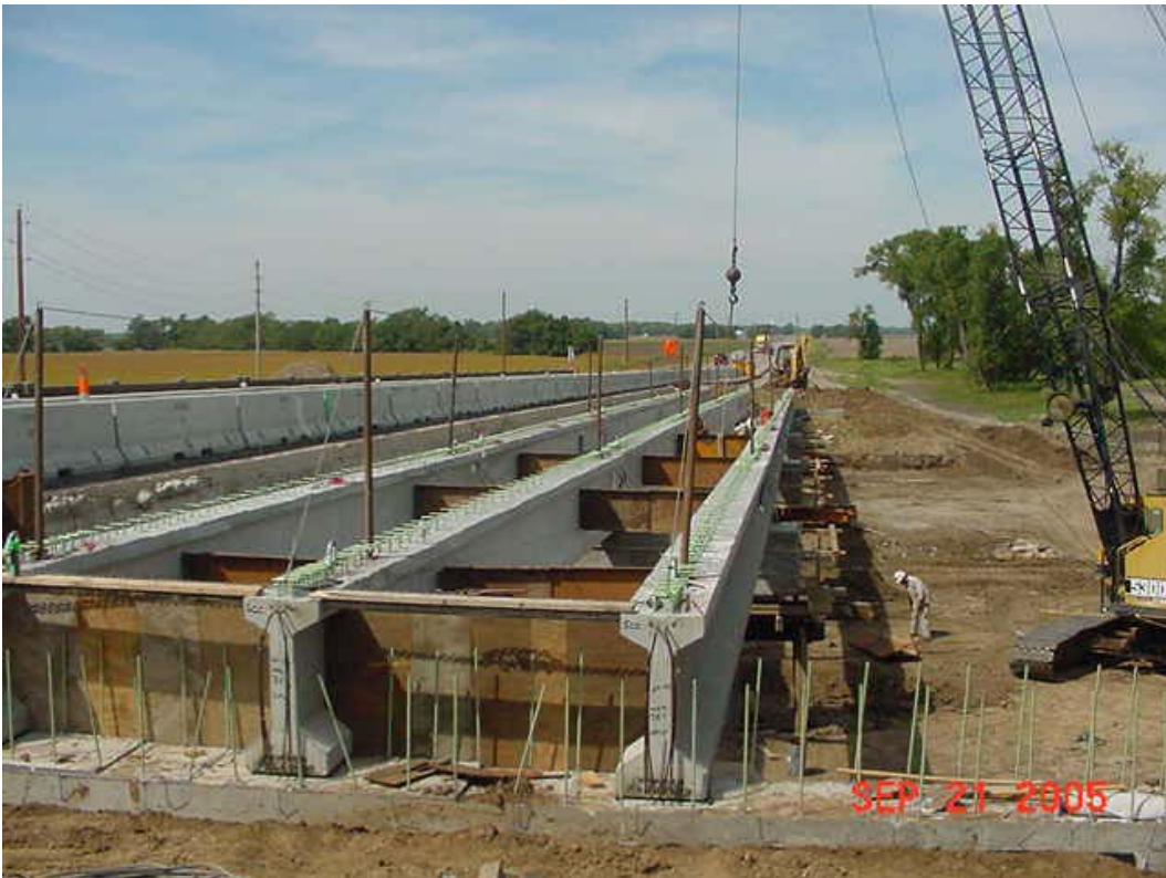
Figure 12.26 Placement of girders
