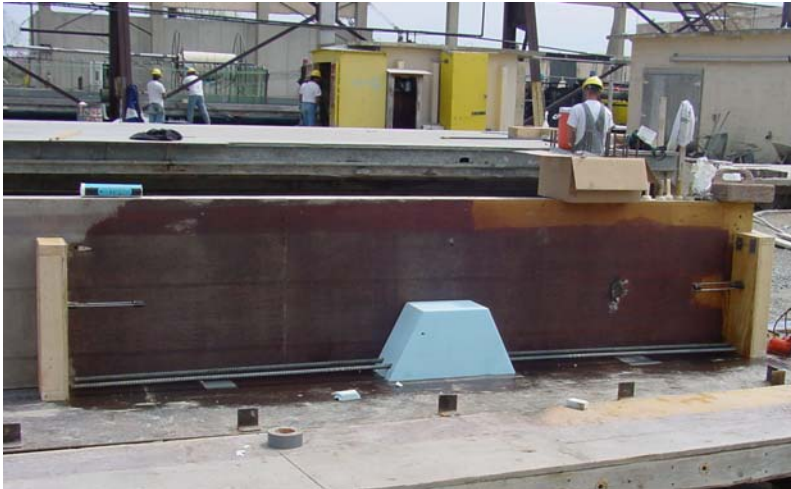
Figure 6.11 Block used to reduce height at mid span
