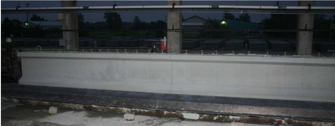
Figure 12.19 Smooth exterior of SCC girder
