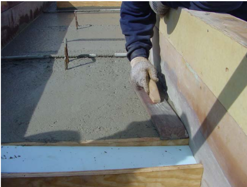
Figure 6.21 Finishing of top surface
