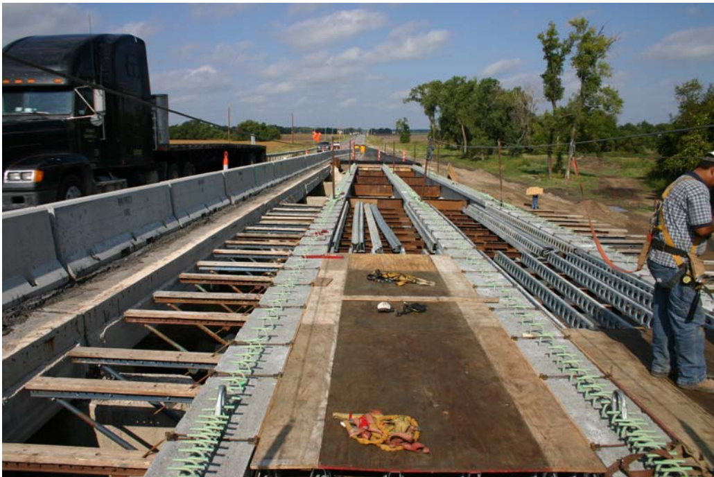
Figure 12.30 Placement of shoring for deck casting-II
