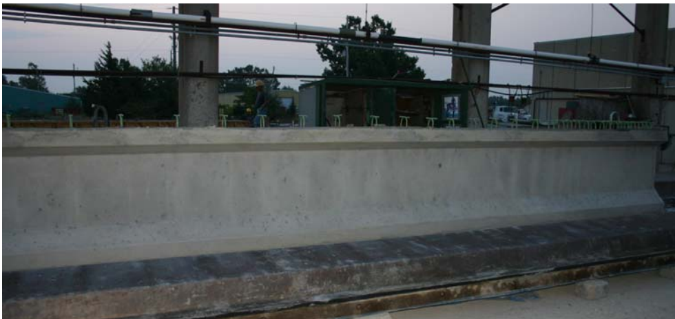
Figure 12.17 Presence of "bug" holes in girder with conventional concrete
