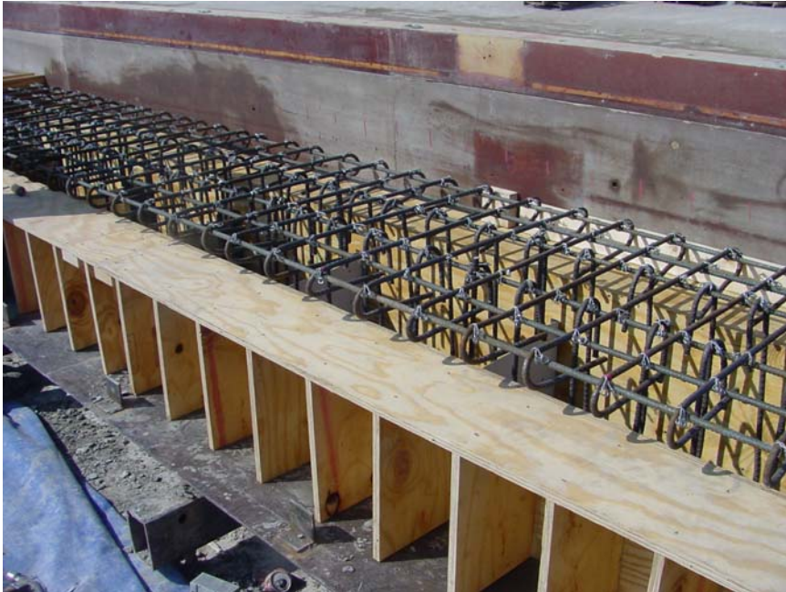
Figure 6.18 Finished shear stirrups in TBs
