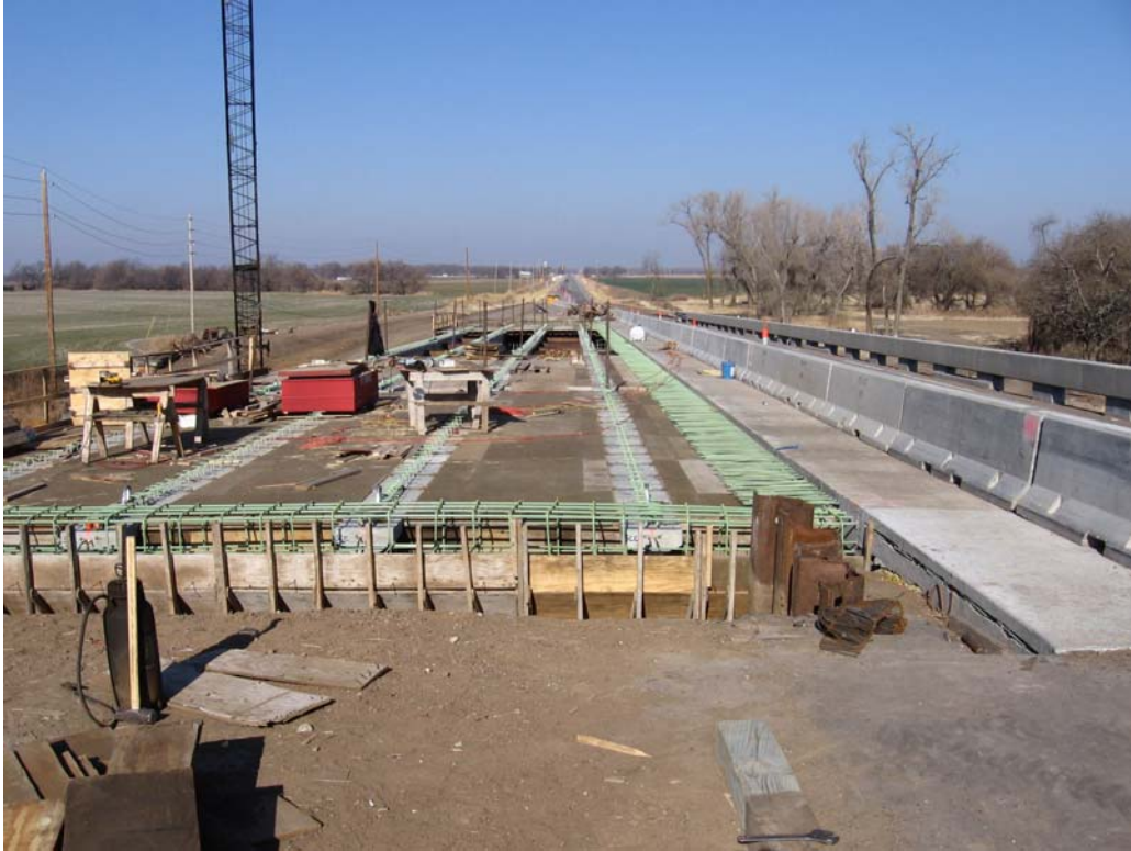
Figure 12.40 Shoring for phase II
