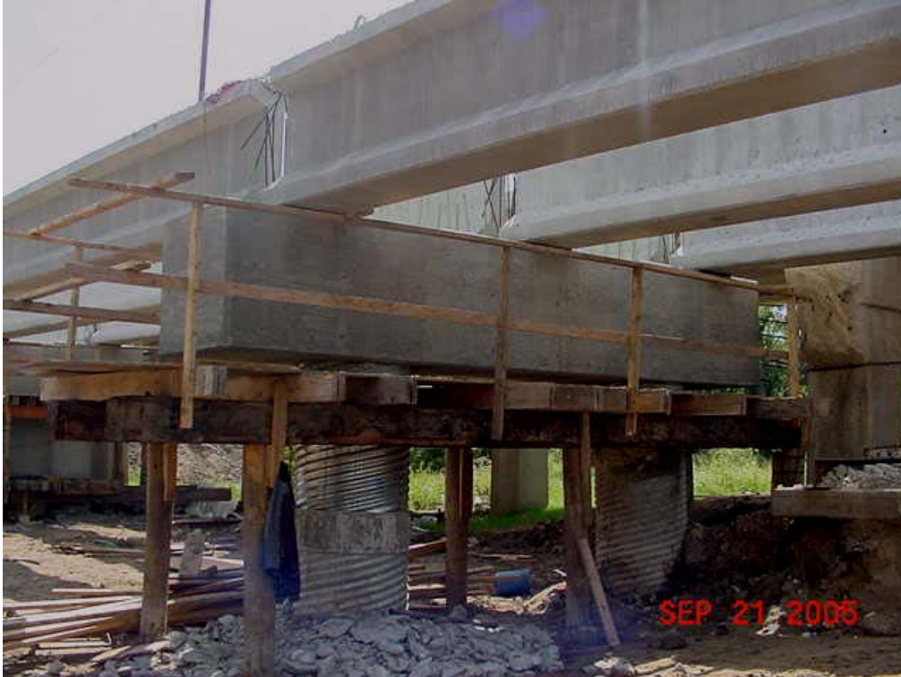
Figure 12.27 Underneath view of placed girders
