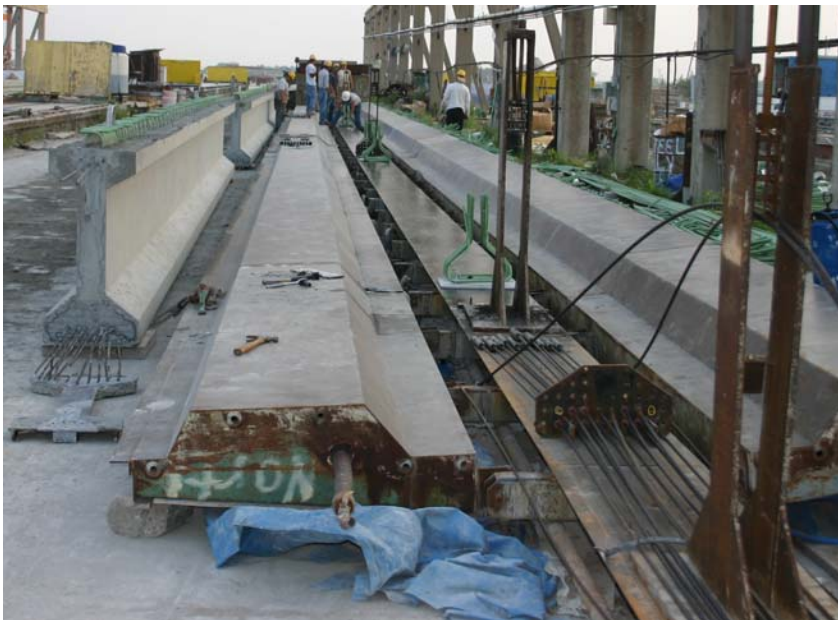
Figure 12.6 Empty prestressing bed
