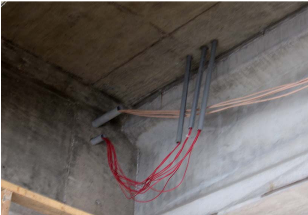
Figure 12.34 Wires extending through abutment wall
