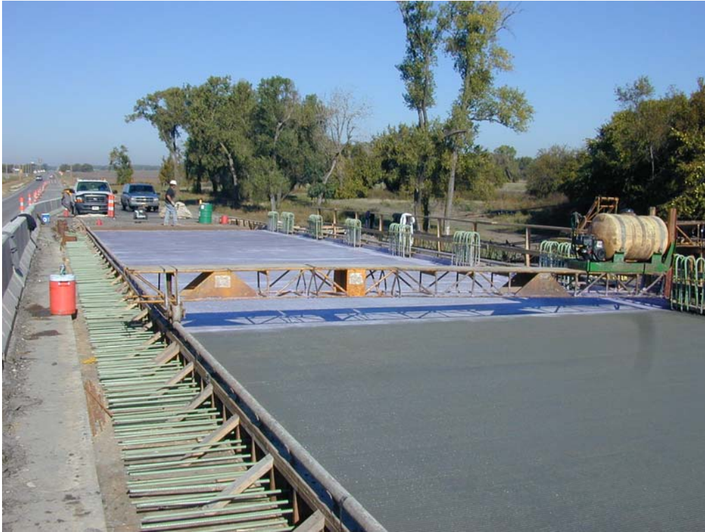
Figure 12.37 Finishing of concrete
