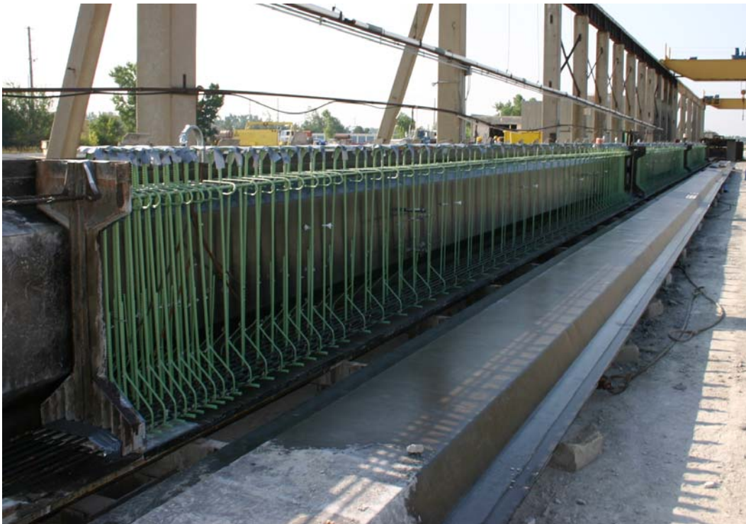
Figure 12.8 Forms after one side wall has been set into place
