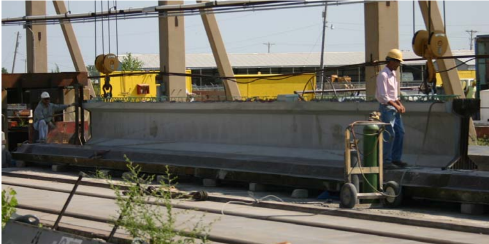
Figure 12.16 Detensioning of strands with a torch
