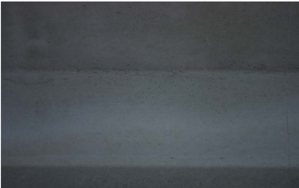
Figure 12.20 Closeup of smooth SCC finish
