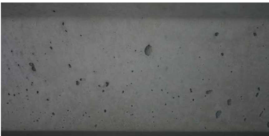
Figure 12.18 Closeup view of "bug" holes in girder with conventional concrete
