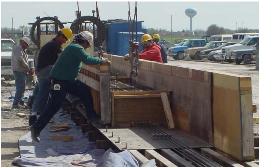
Figure 6.19 Placement of outside walls
