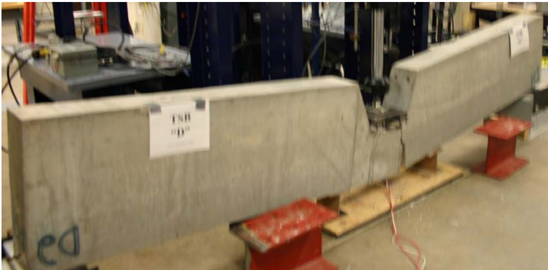
Figure 7.22 Failure of TSB D
