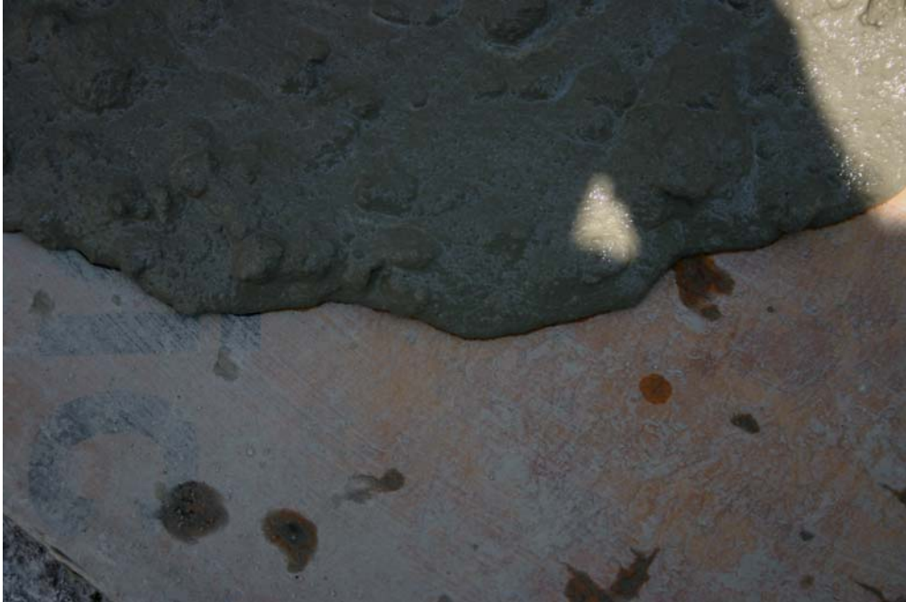
Figure 12.15 SCC mixture showing no excess paste and presence of aggregate on leading edge
