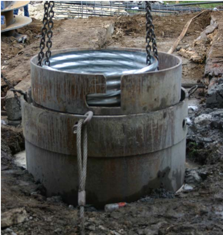
Figure 12.24 Placement of cages for piles
