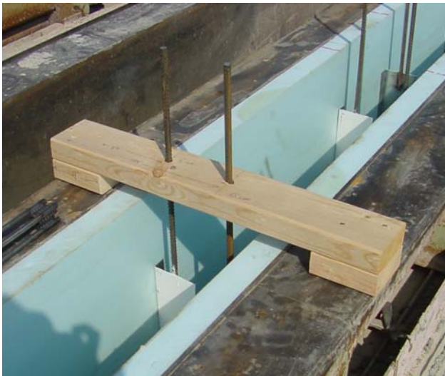
Figure 6.6 Crack former held in with wood 2 x 4
