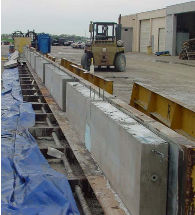
Figure 6.15 Removal of TSB from beds
