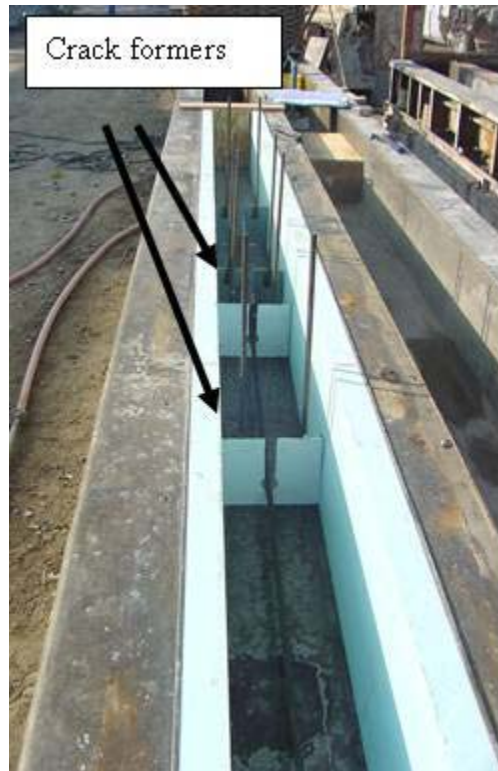
Figure 3.6 Crack former in SSB specimens
