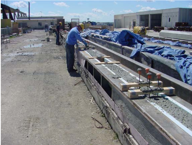
Figure 6.8 Finishing of SSB specimens
