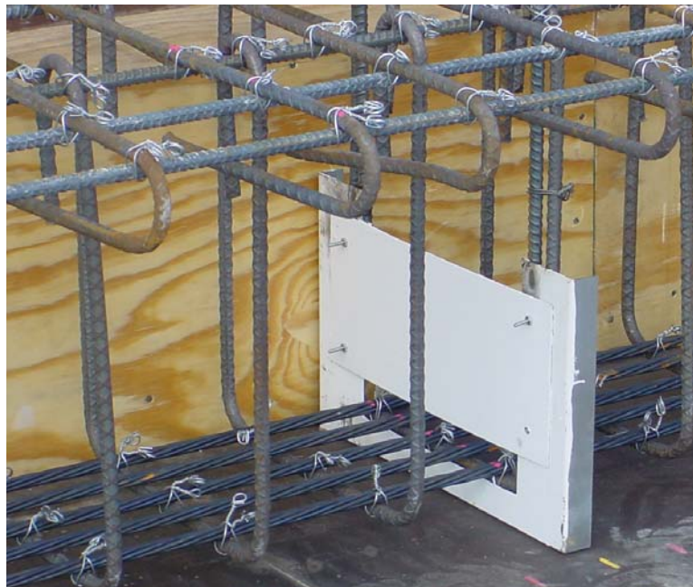
Figure 3.8 Crack former used for TB specimens
