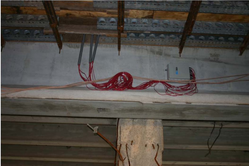
Figure 12.33 Wires extending into multi-plexor
