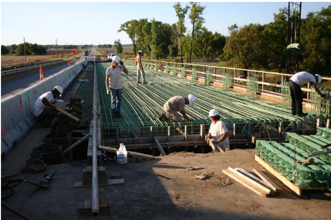
Figure 12.32 Tying of deck reinforcement into place
