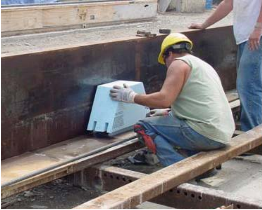
Figure 3.3 Block-out used for top-strand beams
