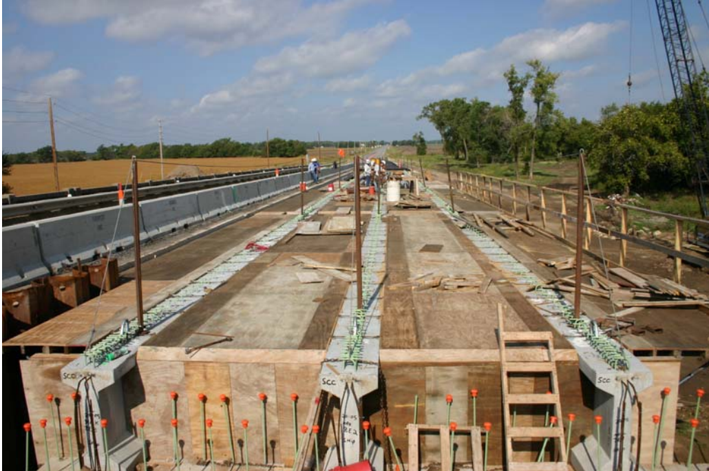
Figure 12.29 Placement of shoring for deck casting
