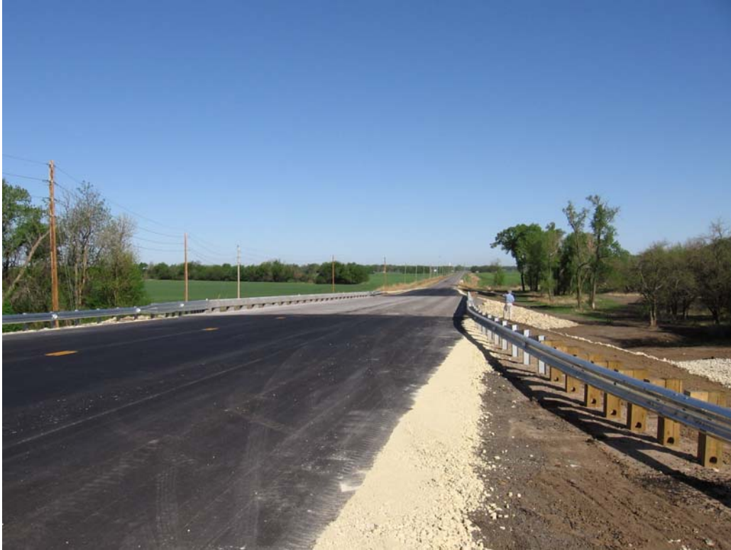
Figure 12.42 Finished bridge and approach
