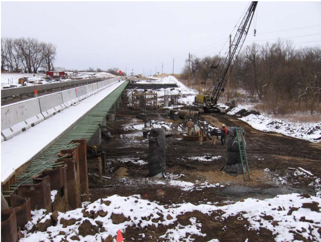
Figure 12.39 Groundwork for phase II
