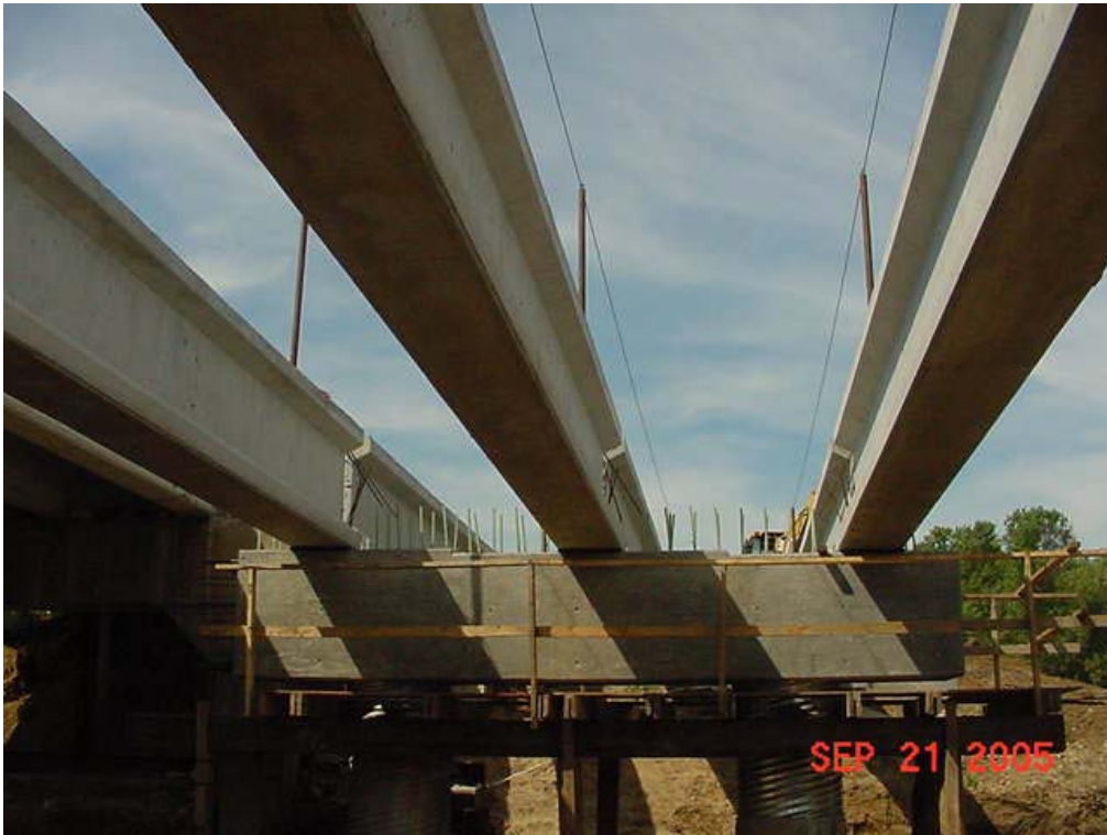
Figure 12.28 Underneath view of placed girders
