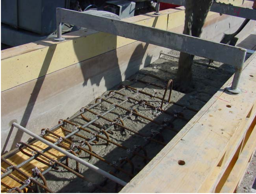
Figure 6.20 Pouring of SCC into forms
