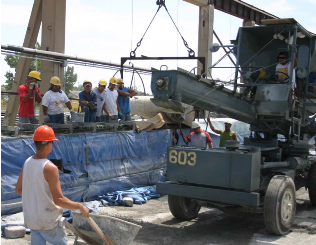
Figure 12.11 Laborers not having to vibrate SCC mixture
