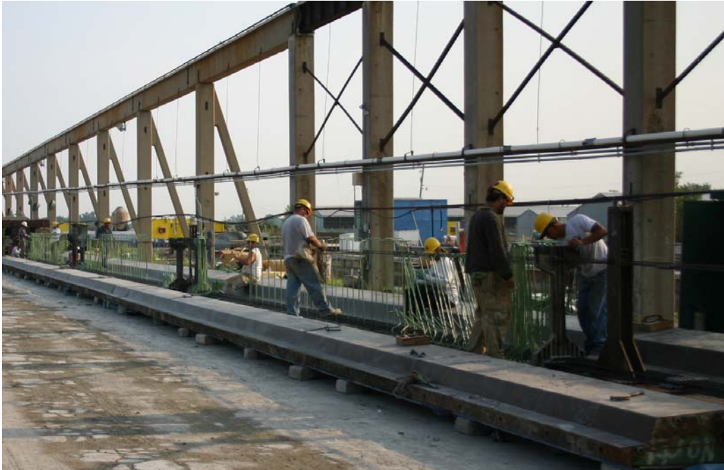
Figure 12.7 Tying of internal shear stirrups
