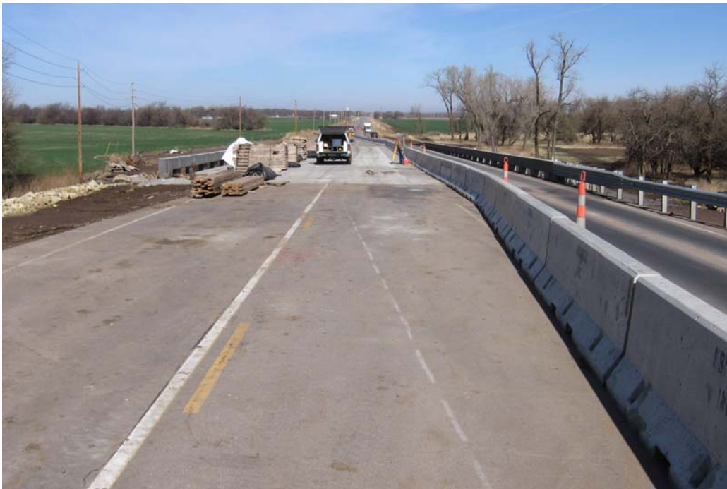
Figure 12.41 Deck completion of phase II
