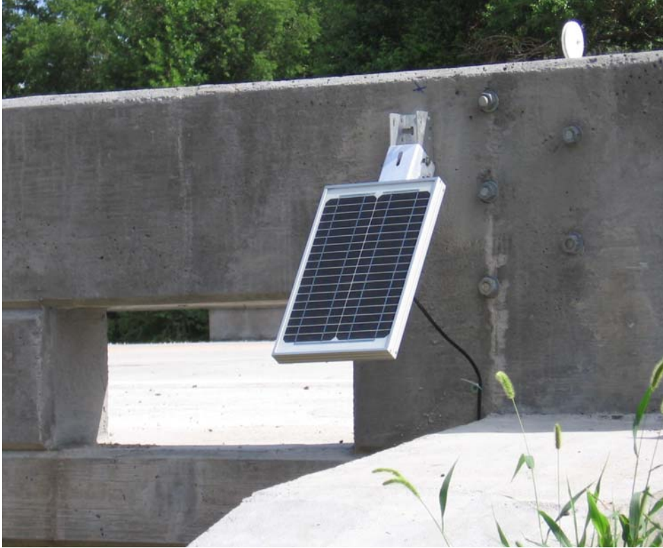
Figure 12.44 Solar panel on side railing
