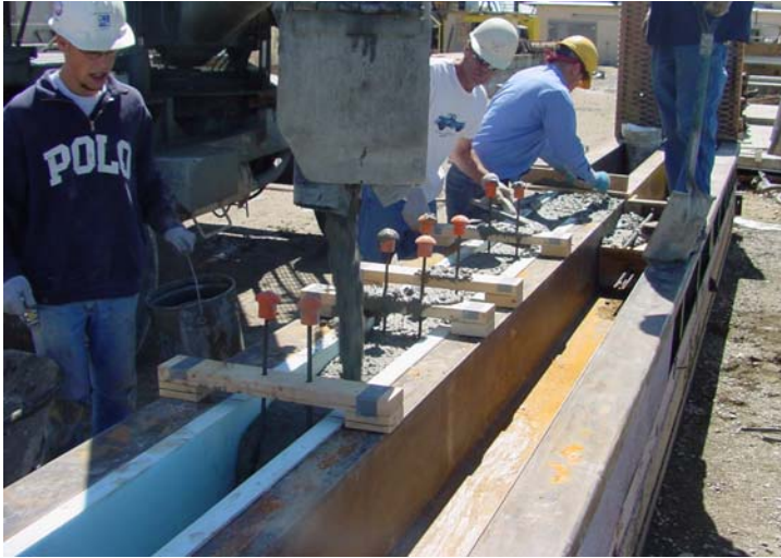
Figure 6.7 Pouring of SCC into forms
