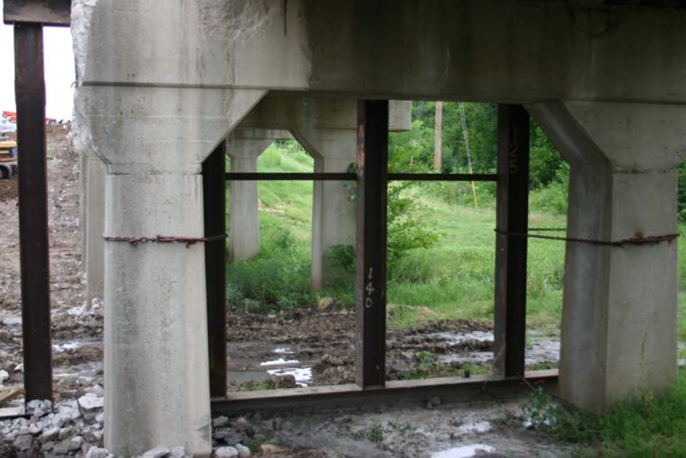
Figure 12.23 Temporary supports for existing bridge
