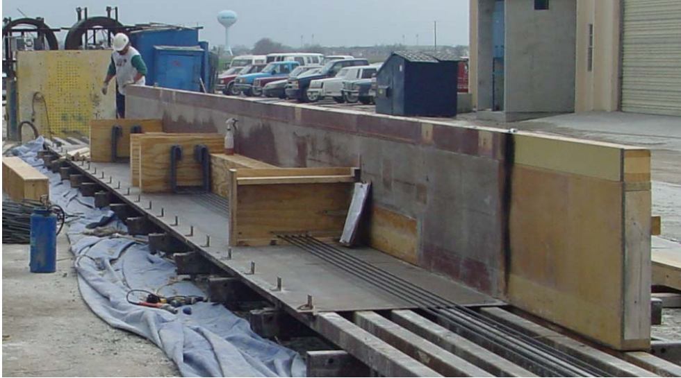
Figure 6.16 Headers spaced for TB specimens
