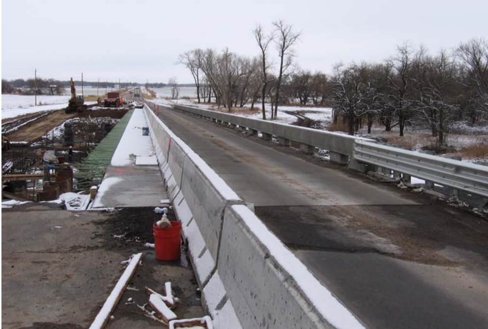
Figure 12.38 Opened lane of phase I and beginning of phase II
