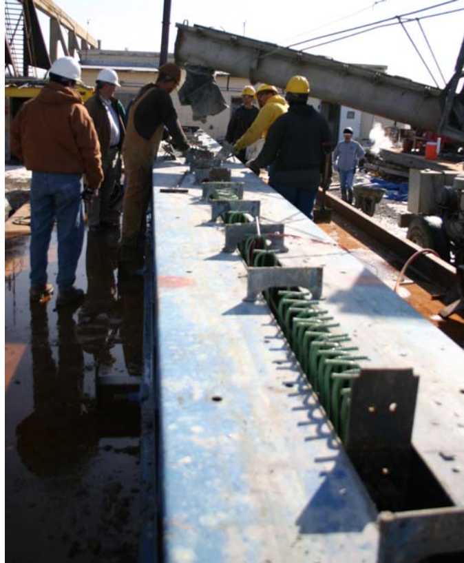
Figure 8.8 Placement of SCC
