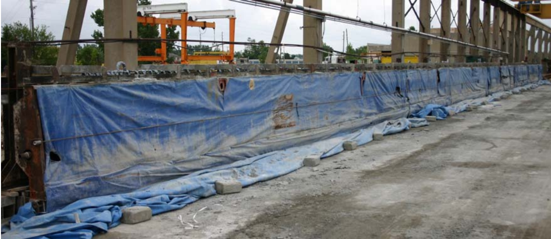
Figure 12.9 Prestressing bed after walls have been set into place
