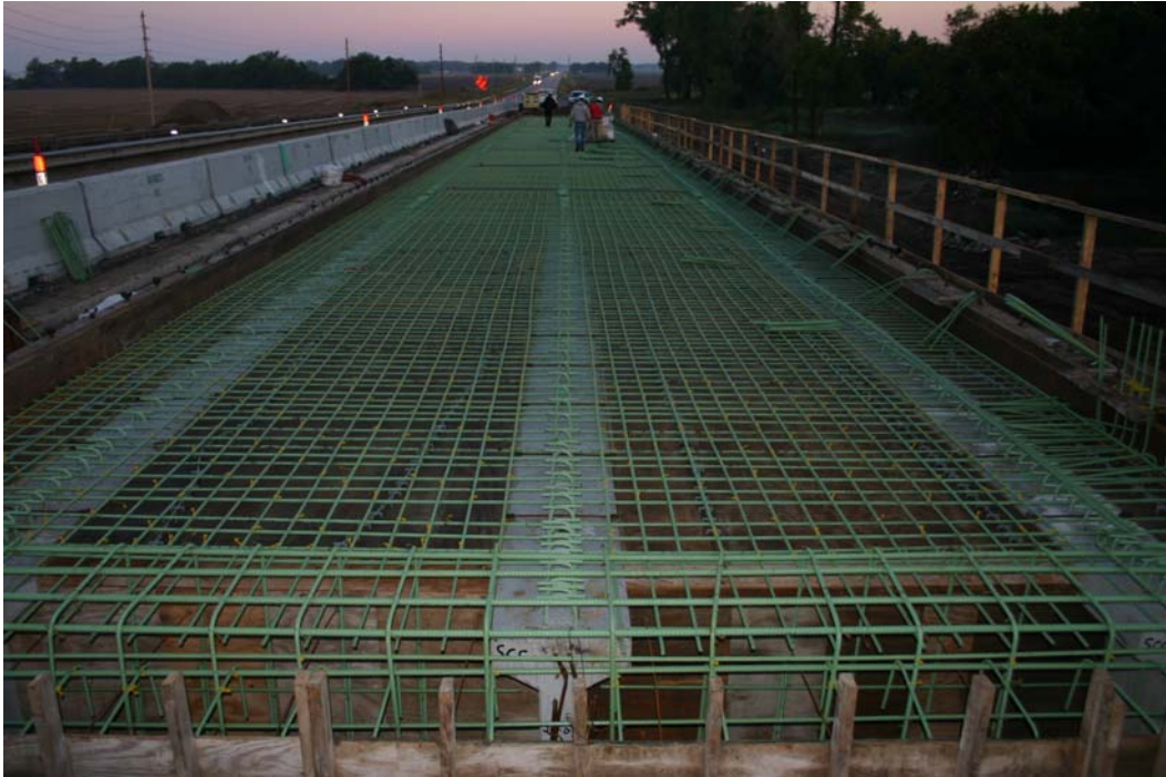
Figure 12.31 Placement of deck reinforcement
