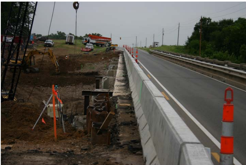
Figure 12.22 One lane open to traffic during phase I construction
