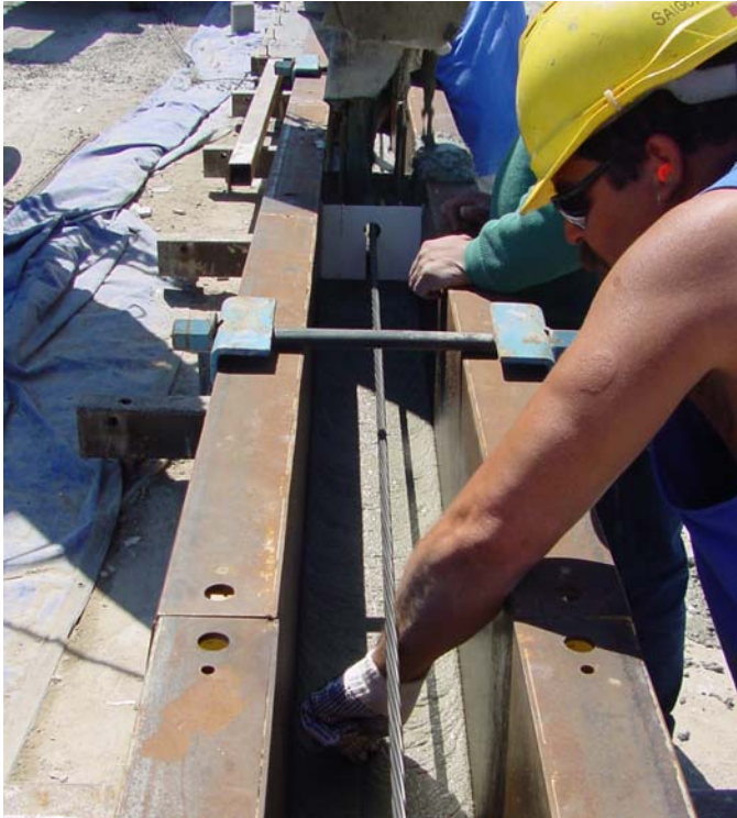
Figure 6.13 Pouring of SCC into forms
