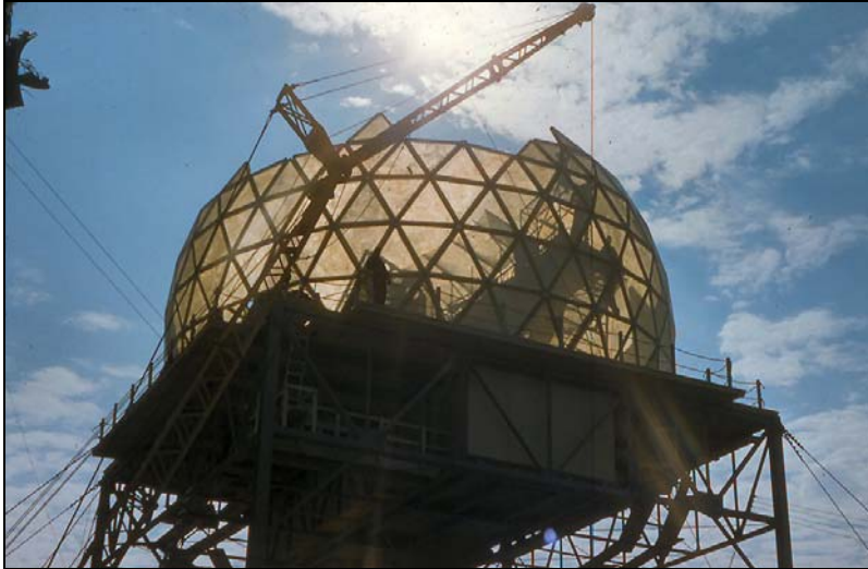
Figure 8.2 A radome under construction on the DEW Line ( http://www.porticus.org/bell/images/ollie/ollie27.jpg )
