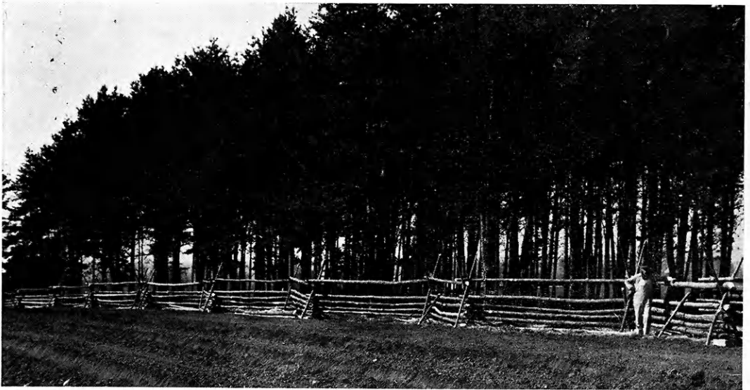
THE PINE POLE FENCE RECENTLY CONSTRUCTED ALONG THE OLD HORT PINE GROVE
