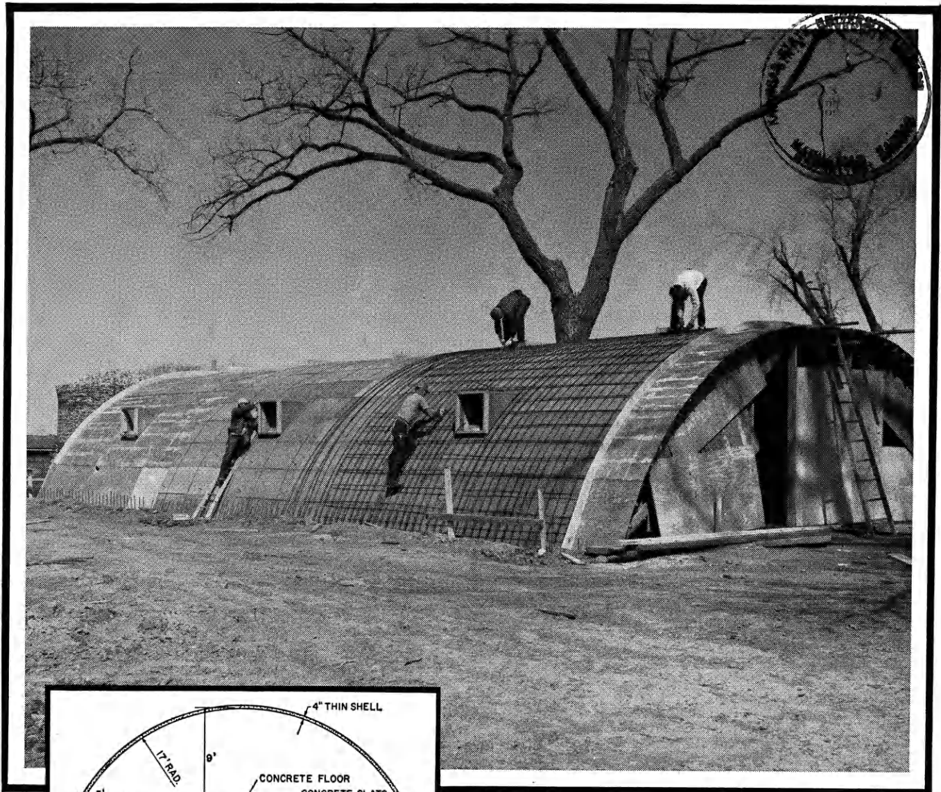
Concrete thin-shell hog house under construction showing (left to right) plywood forms, polystyrene insulation and reinforcing bars.
