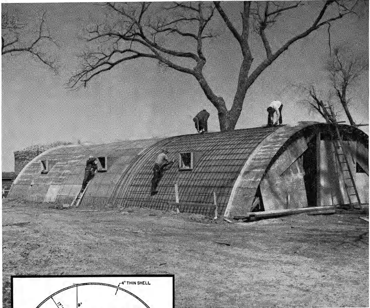
Concrete thin-shell hog house under construction shown (left to right) plywood forms, polystyrene insulation and reinforcing bars.
