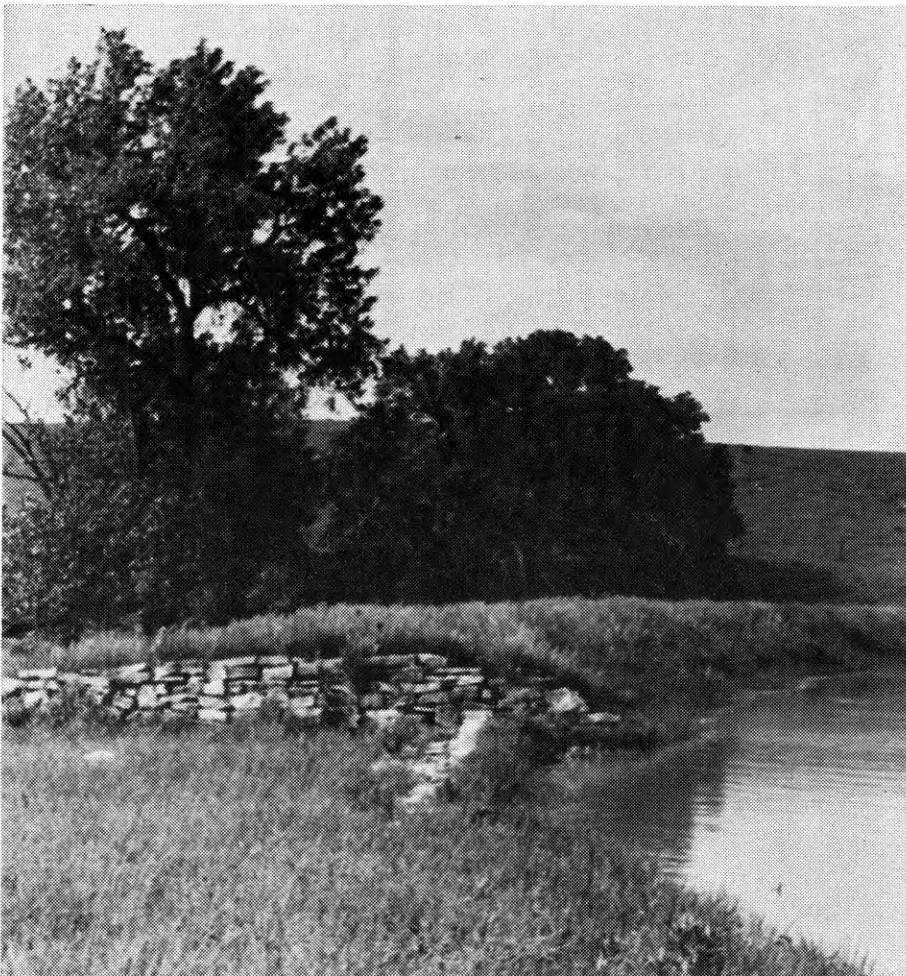
This pond is built correctly. Rocks in spillway and grass on dam prevent washing.
