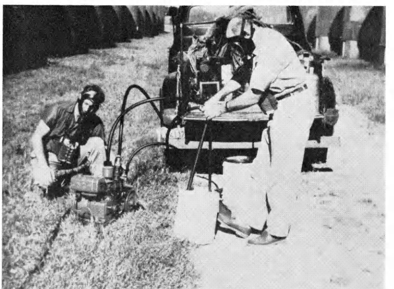
A storage bin should be sealed to reduce the loss of fumigant chemicals. A compact spraying unit can be carried in the back of a pick-up truck.
