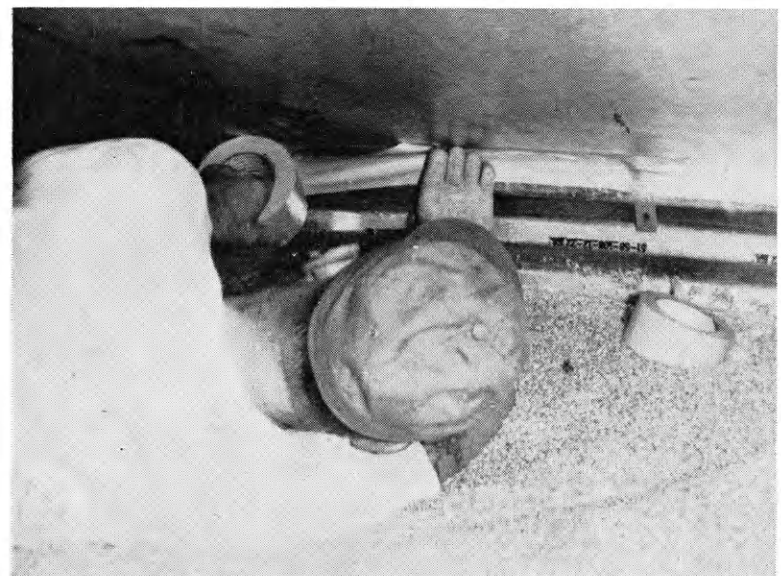
A storage bin should be sealed to reduce the loss of fumigant chemicals. A compact spraying unit can be carried in the back of a pick-up truck.
