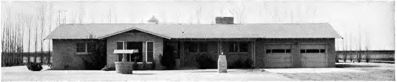
Concrete masonry home of Mr. and Mrs. Earl Greene, Plainview, Texas
