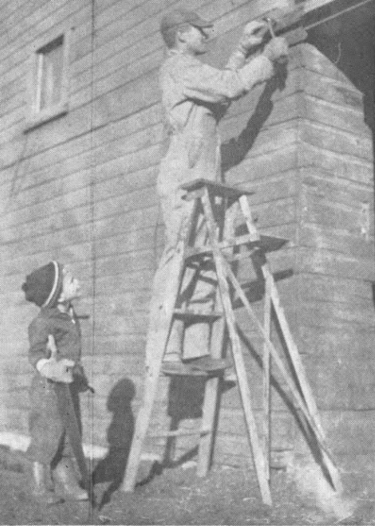
Check and repair your barn carefully. A two-story barn like this would cost about four dollars per square foot of floor space to replace. Repairing buildings pays well.
