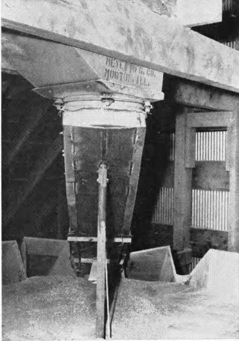
The elevator chute is on a spindle so it can be revolved to empty in any of the bin chutes.
