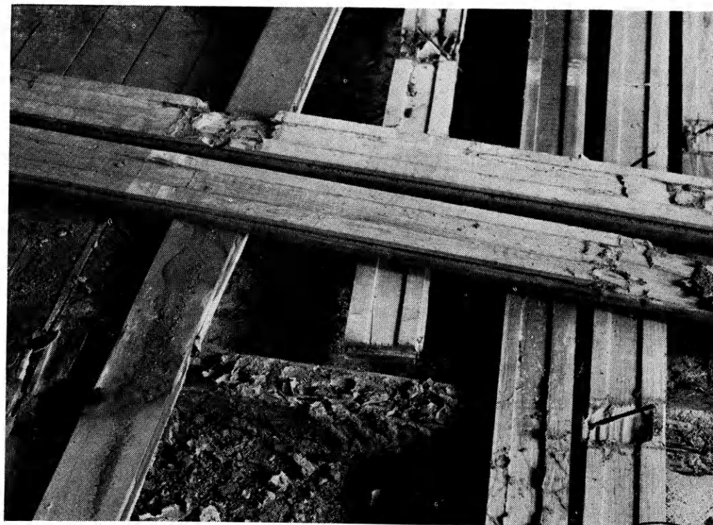
THIS IS WHAT happens when the floor supports touch the soil. The insects eat the insides from floor boards leaving only paper-like hulls, which are unsafe. Proper repair of floors and foundations and proper spraying with Chlorodane will usually eliminate the nests.
