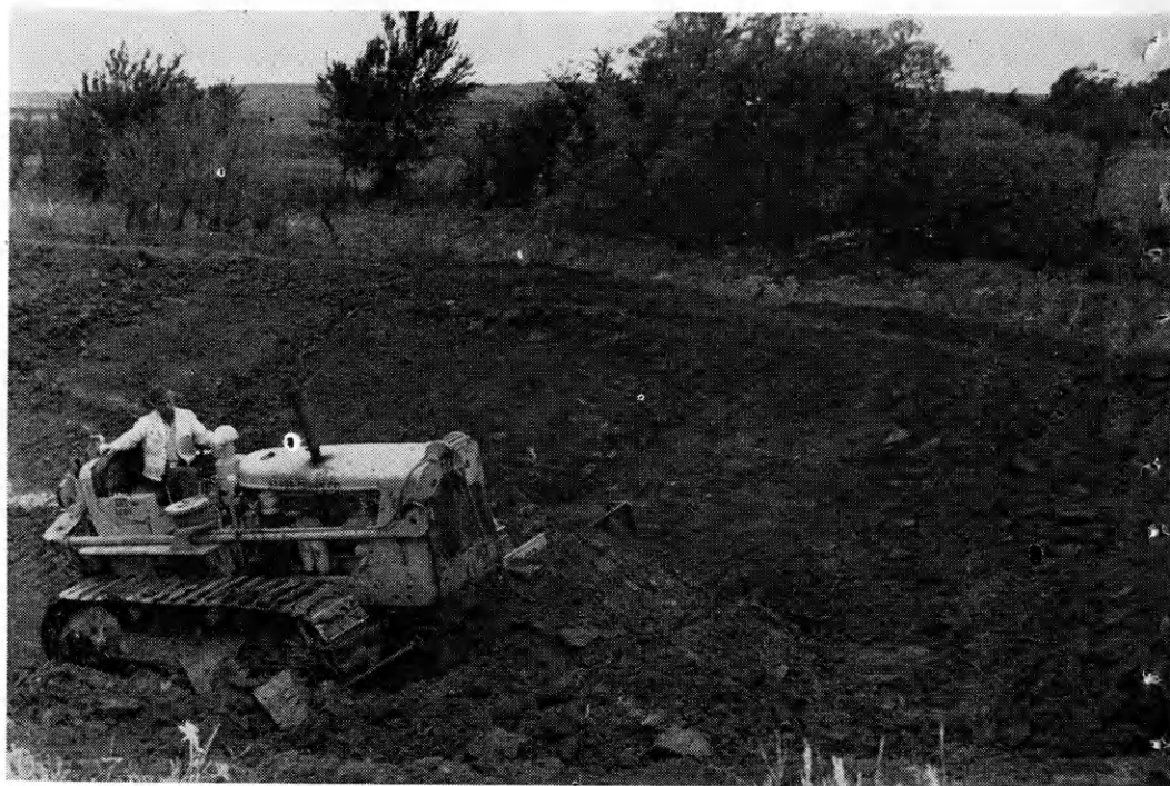
A NEW ANGLE is to dig a reservoir to store water from irrigation wells. Then use it to supplement the wells during hot, dry spells when they won't pump fast enough.
