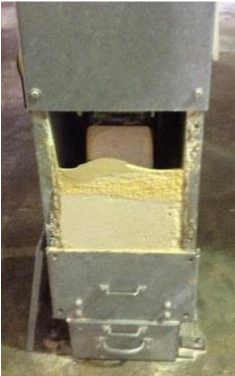
Figure 1.6 Bucket elevator with potential contamination
