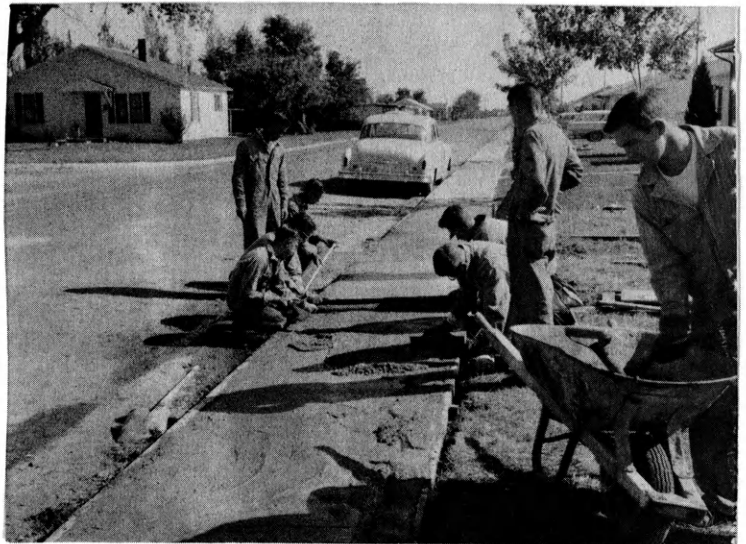
The Plainville Sophomore Ag. class are "learning by doing." The class formed, poured and finished this 150 feet of sidewalk as part of a unit in concrete work.
