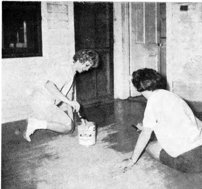
Two coeds wield brushes in painting the porch of the main lodge at the Ranch. Several building interiors were also painted.
