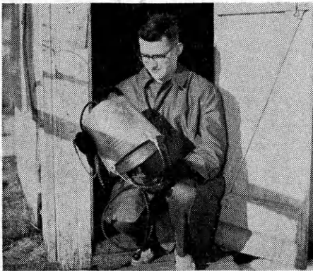
FOR HIS POULTRY PROJECT James made this electric brooder by installing a heat lamp in the bottom of a bucket to provide warmth for baby chicks.
