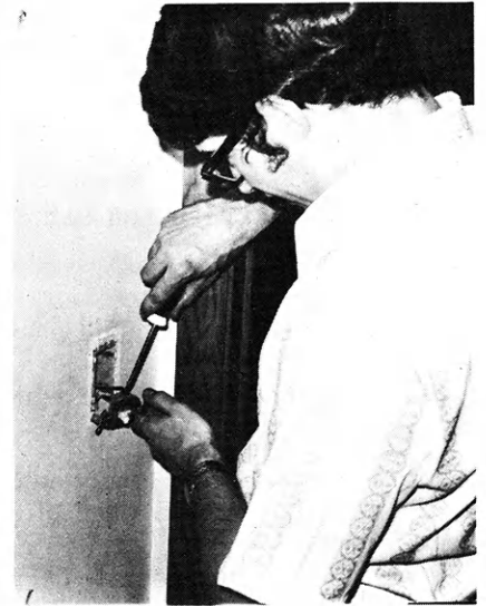
In place of an ordinary light switch, Brent installs a hi-lo dimmer switch.
