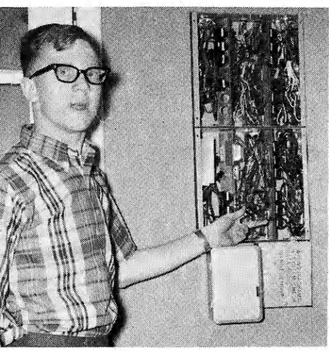
Showing the low voltage "Remote Control Relay Center" in the new Pattinson home, Jim tells how he helped his father with the wiring.
