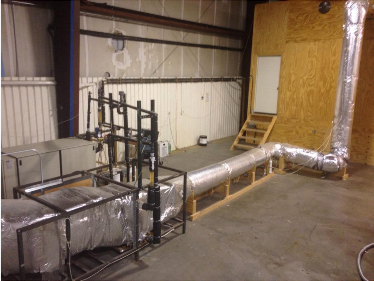
Figure 3.9: Air Supply Ductwork
