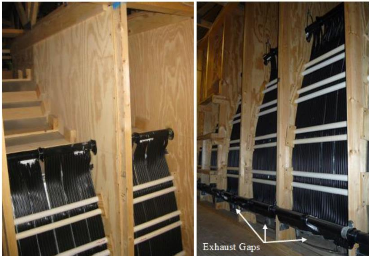
Figure 3.3: Cabin Supports and Exhaust Gaps (Trupka, 2011)
