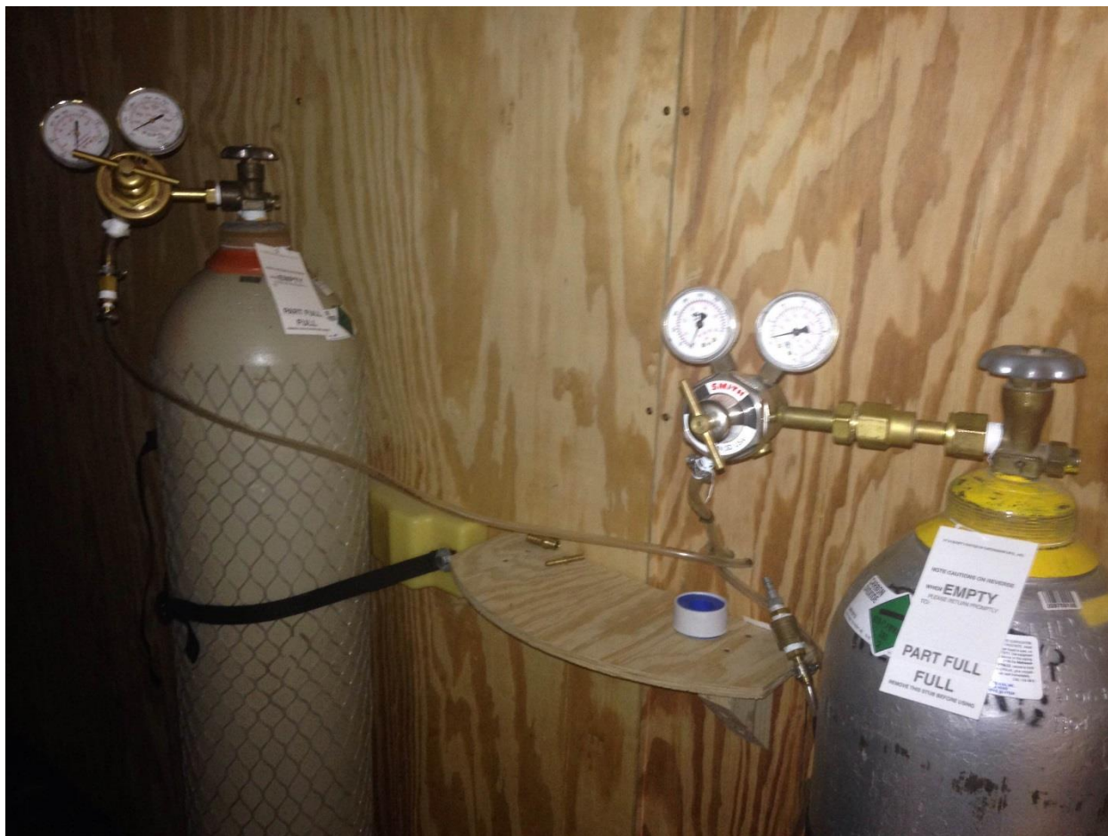
Figure 3.15: Gas Cylinders with Regulators
